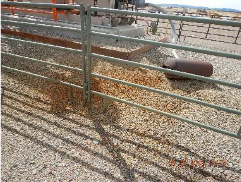
Photo 3: Impacted gravel at muffler exhaust..
