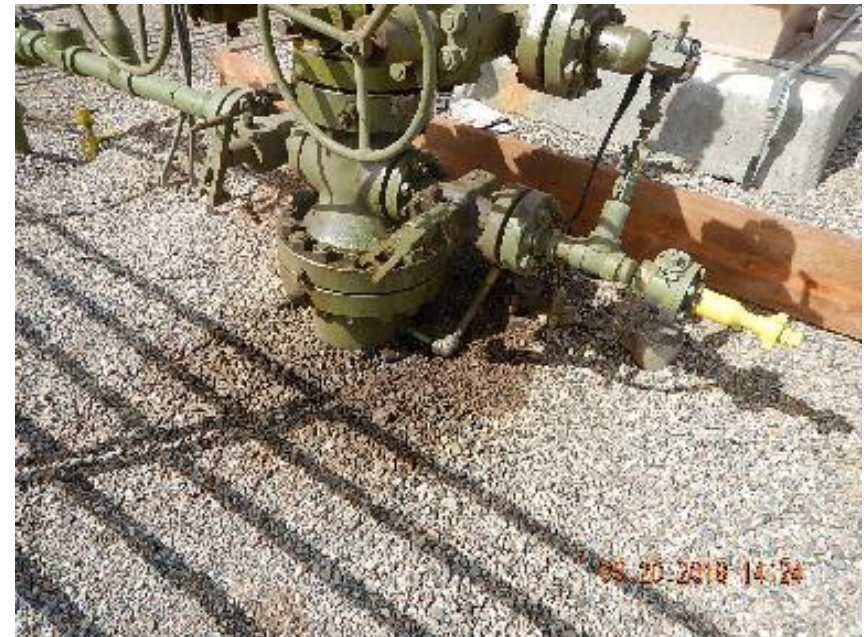
Photo 2: Impacted gravel at wellhead.
