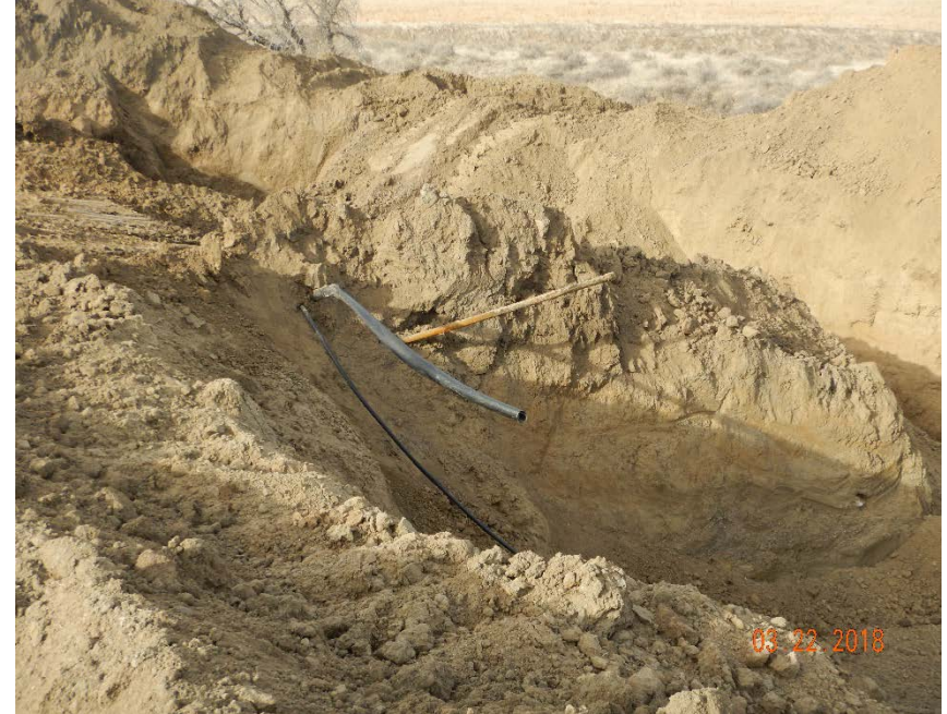
Photo #2 – Exposed flowlines inside of historical release excavation.
