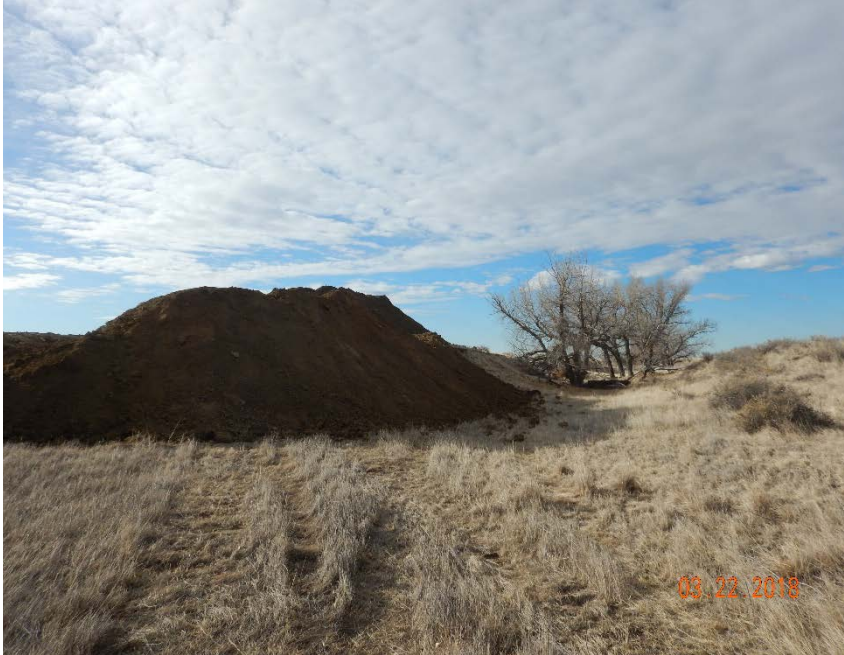
Photo #3 – View from north of stockpiled soil encroaching into adjacent drainage. Note absence of stormwater BMPs.
