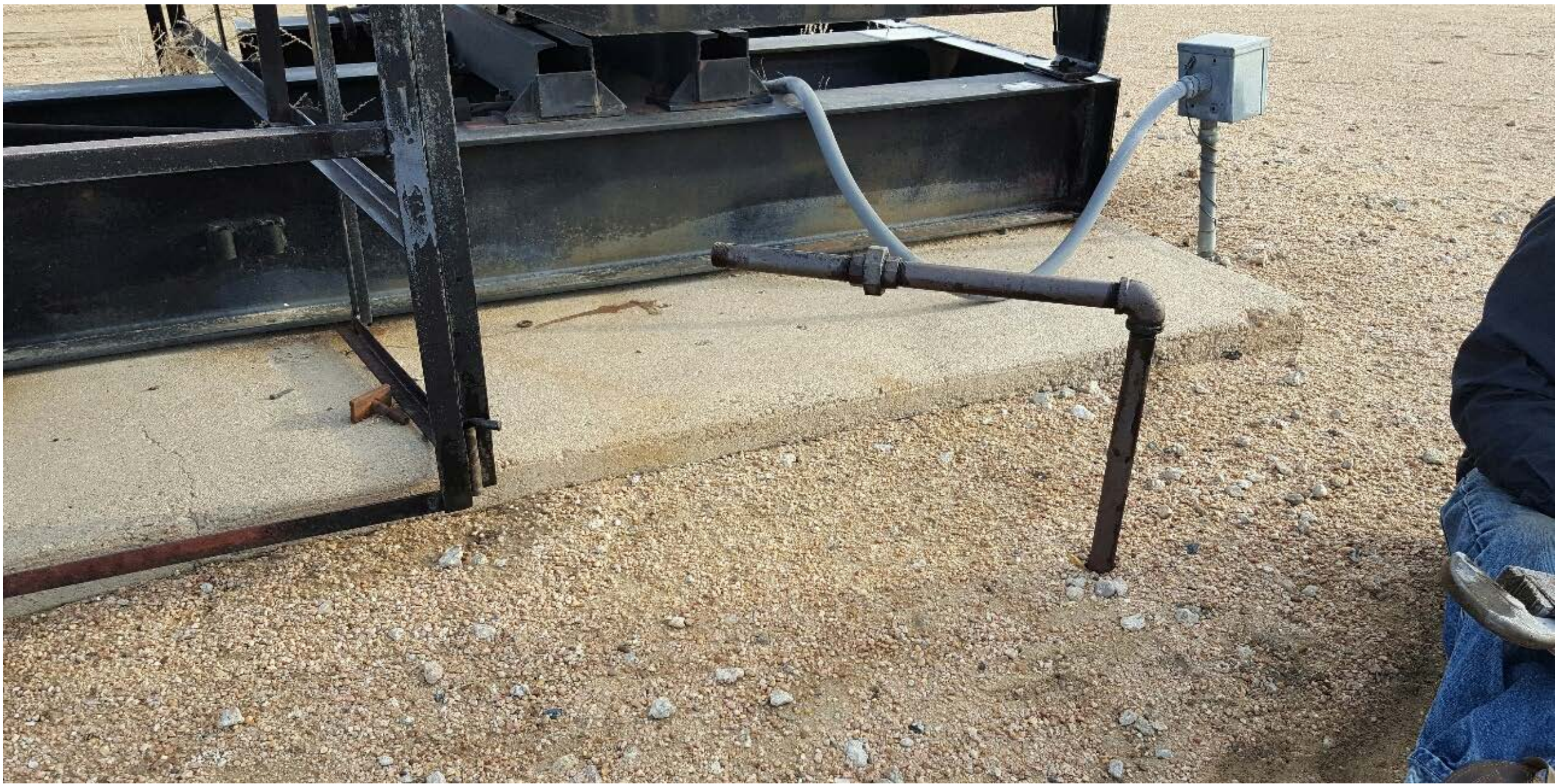
Figure #1 Unmarked riser.
