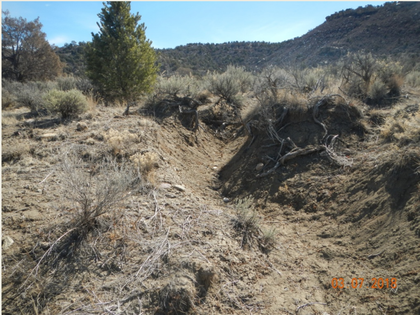
Photo 3. View of erosional channels in the southeastern portion of the project area where concentrated stormwater flows have eroded the cut-slope. Stormwater controls are needed to stabilize erosion here.
