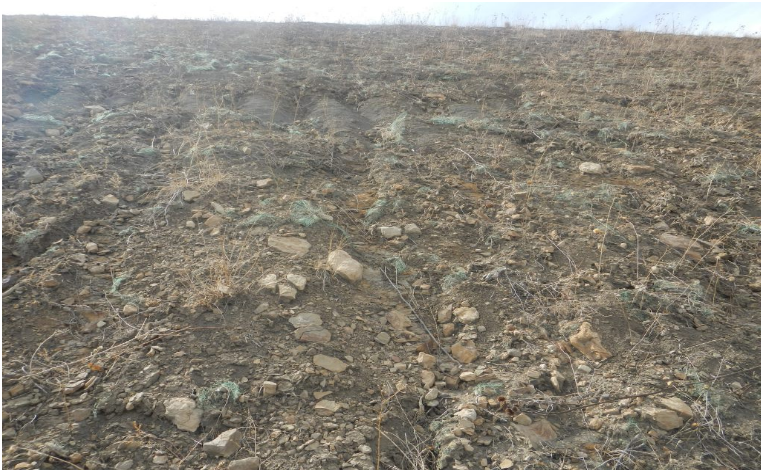
Photo#2: Rill erosion is occurring on Cut Slopes.
