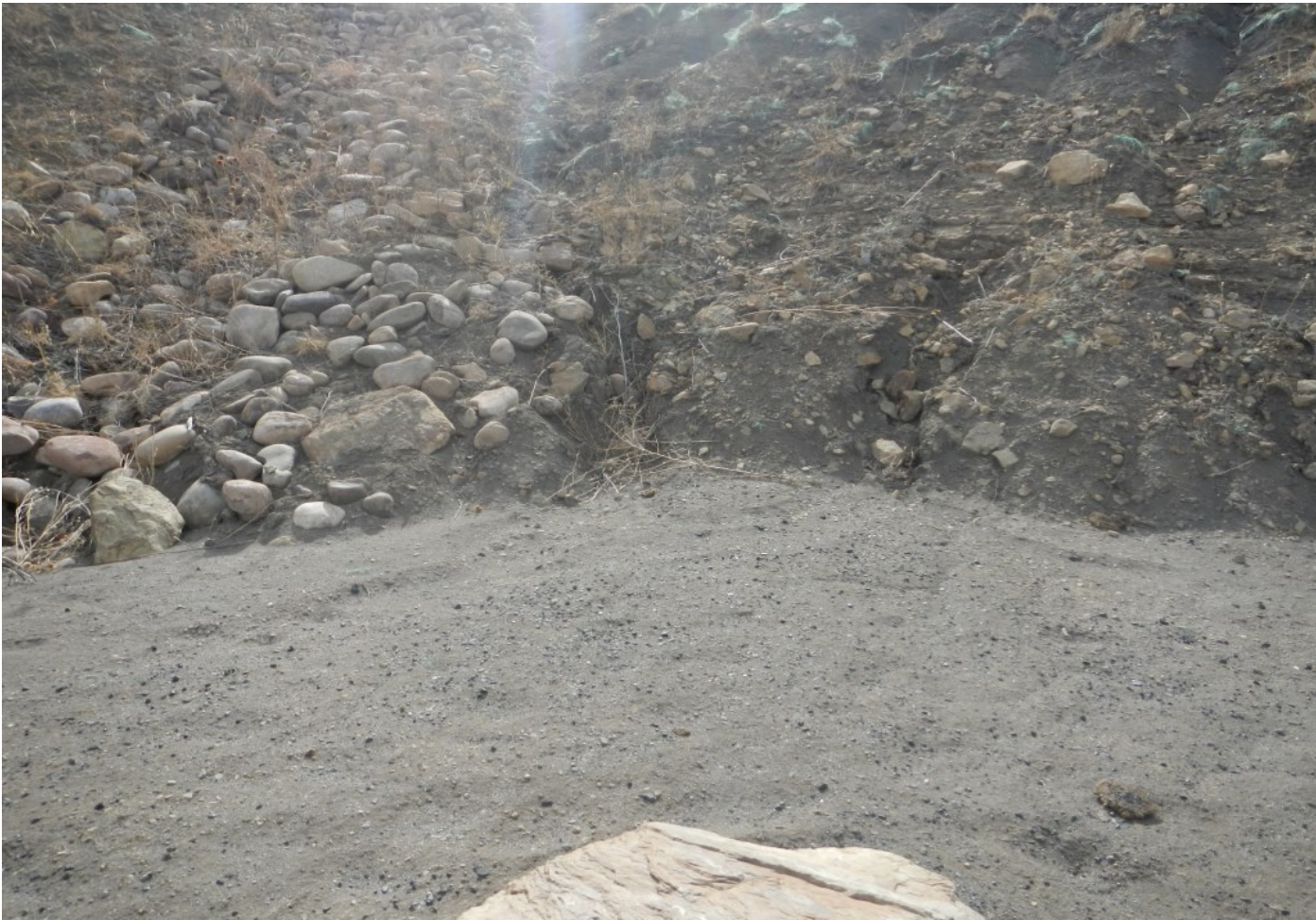
Photo#4: Sediment is still migrating off Cut Slope.
