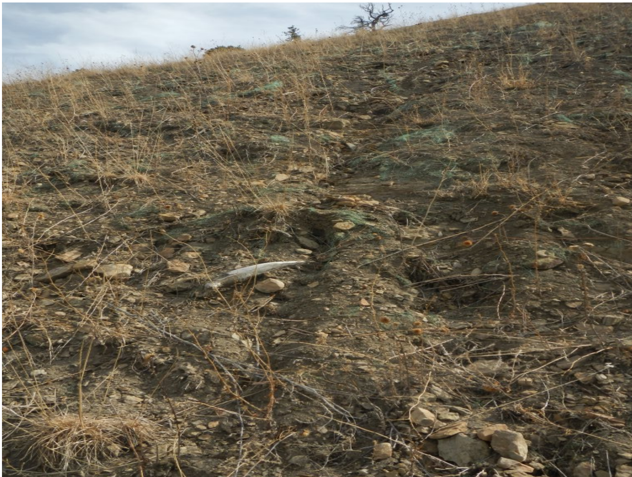
Photo#3: Rill erosion is occurring on Cut Slope .
