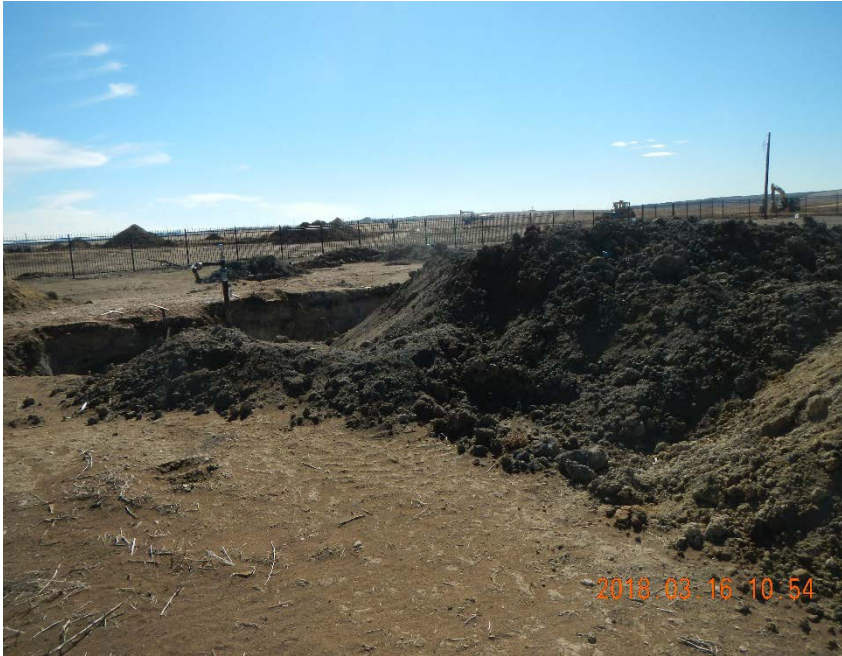
Spoil piles of excavated soil with no storm water BMPs
