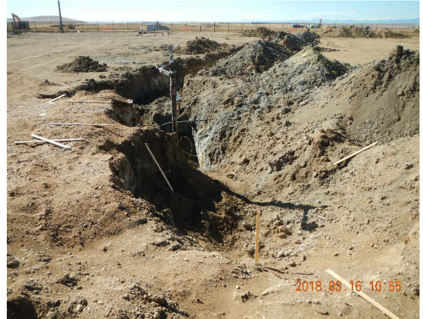
Spoil piles without storm water BMPs
