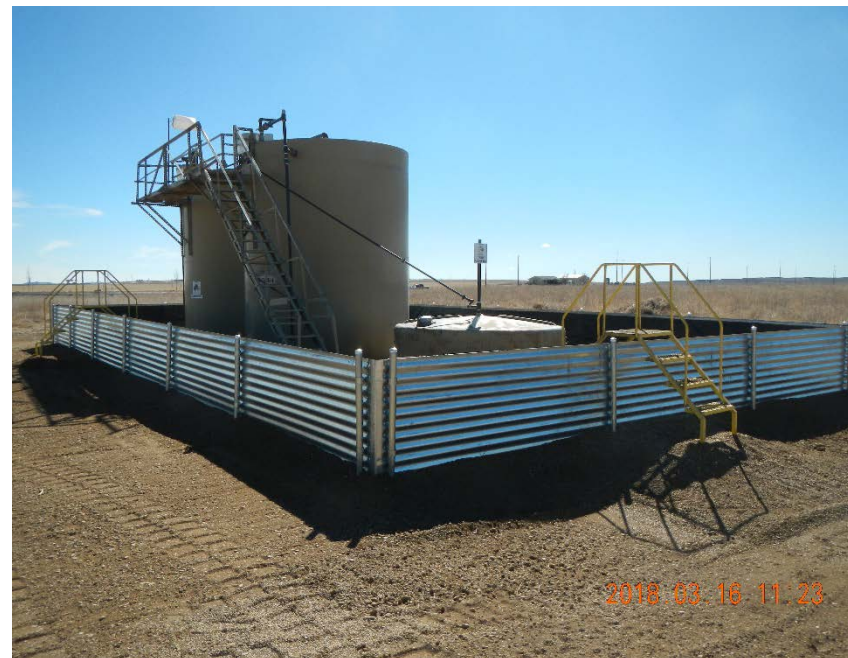
Recently constructed tank battery at the wellhead. Operator has replaced earthen berms with a steel berm.
