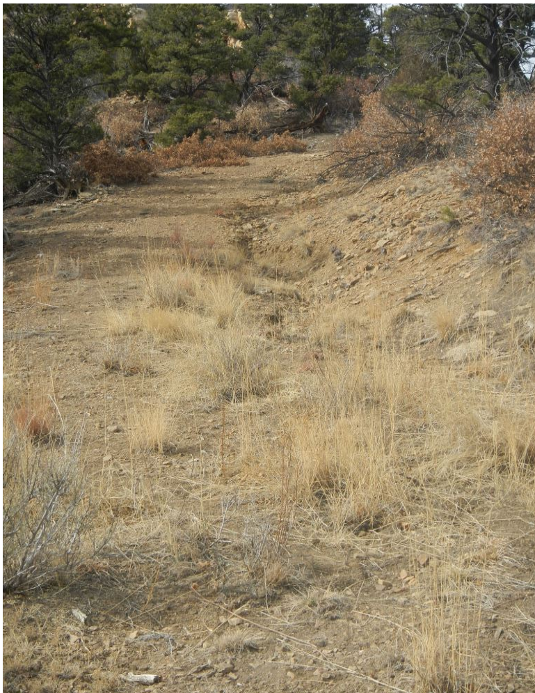
Photo#4: Erosion is occurring on Access Rd.
