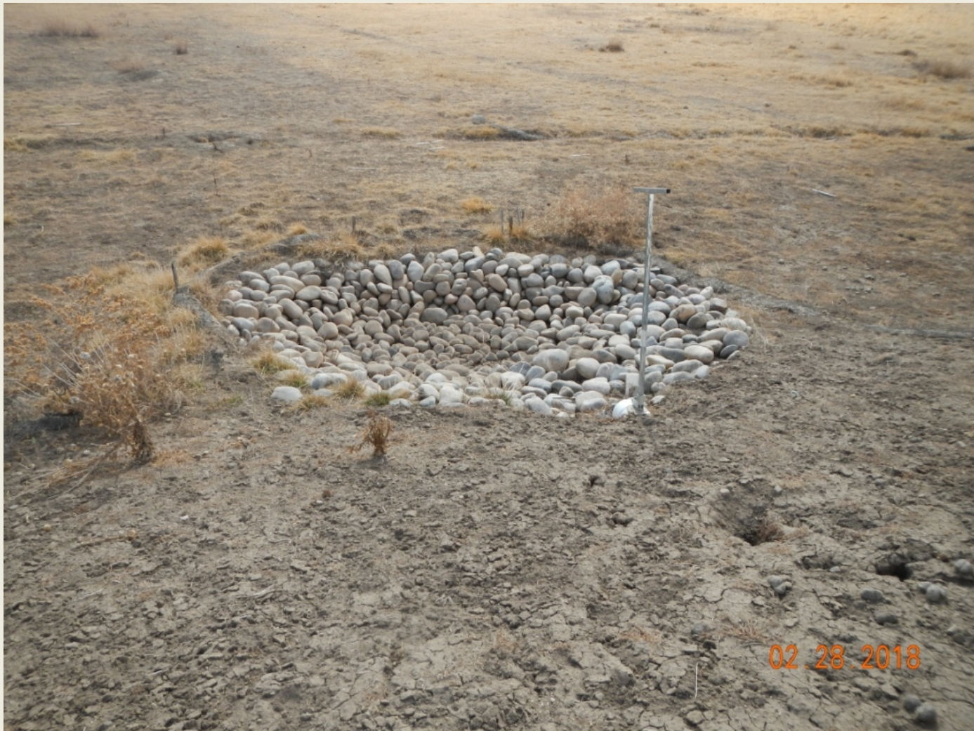
Photo 5. View of silt trap in the southern portion of the project area, appears to be functioning.
