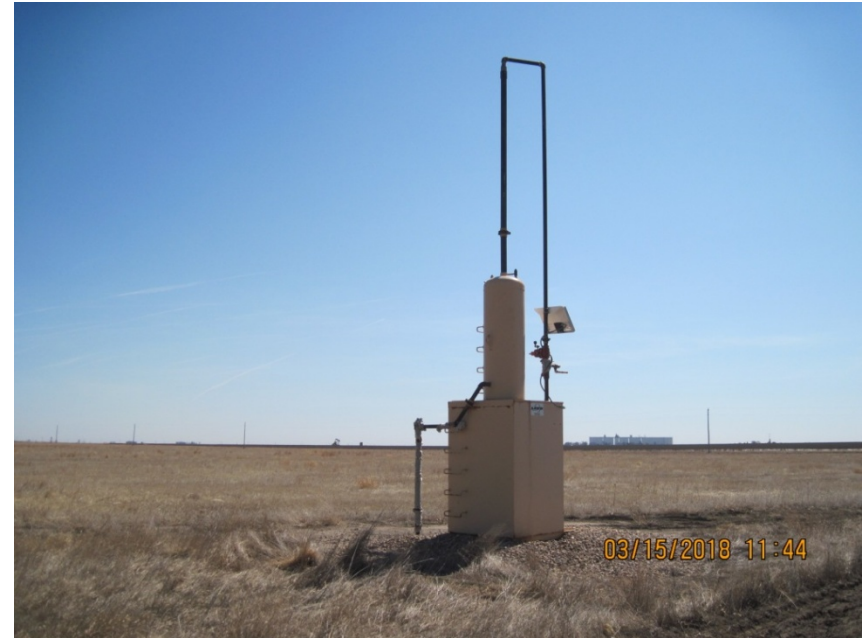
2. Meter shed with vertical gas separator
