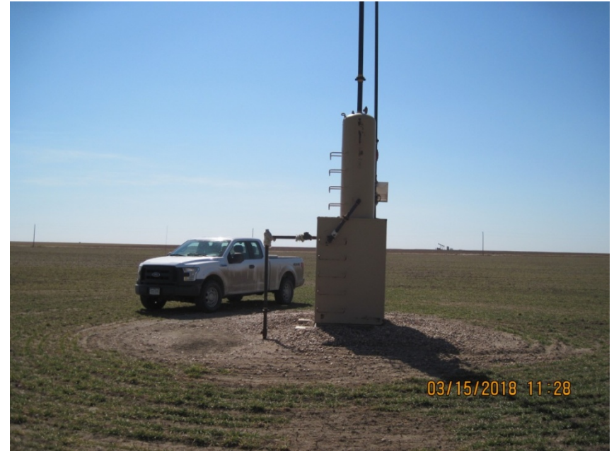
2. Meter shed with vertical gas separator
