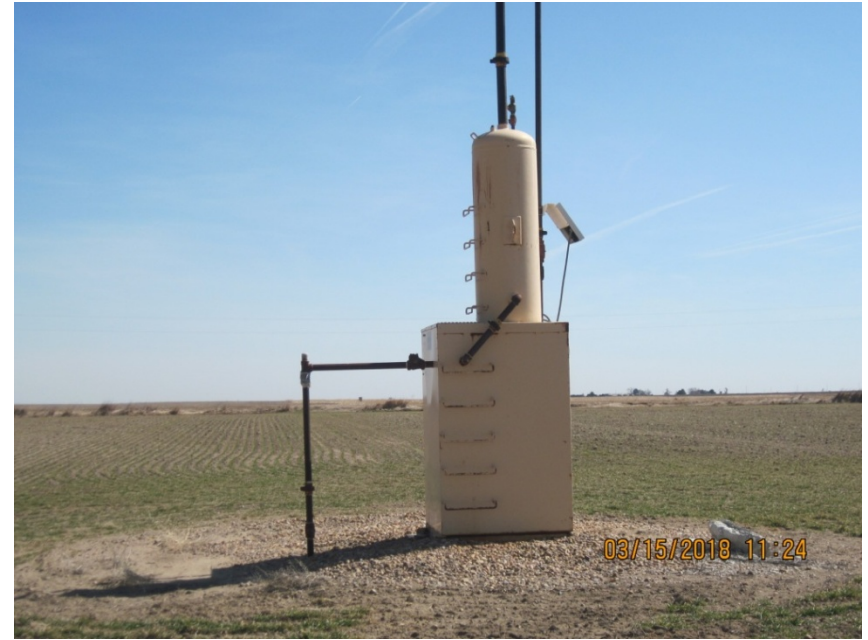
2. Meter shed with vertical gas separator
