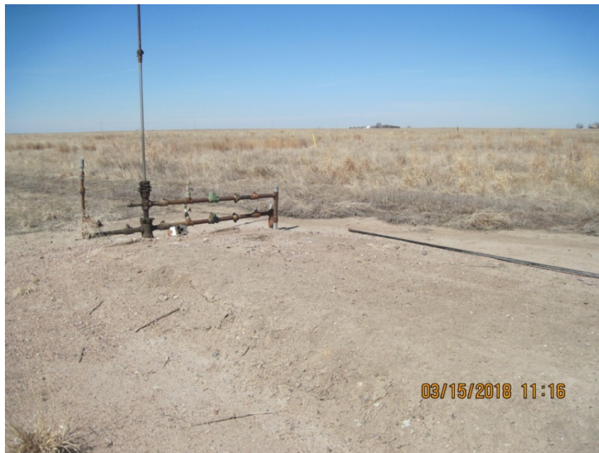
3. Wellhead equipment has been removed
