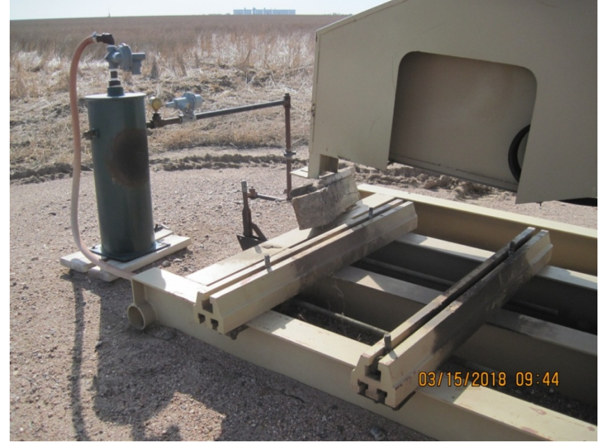
4. Prime mover has been removed
