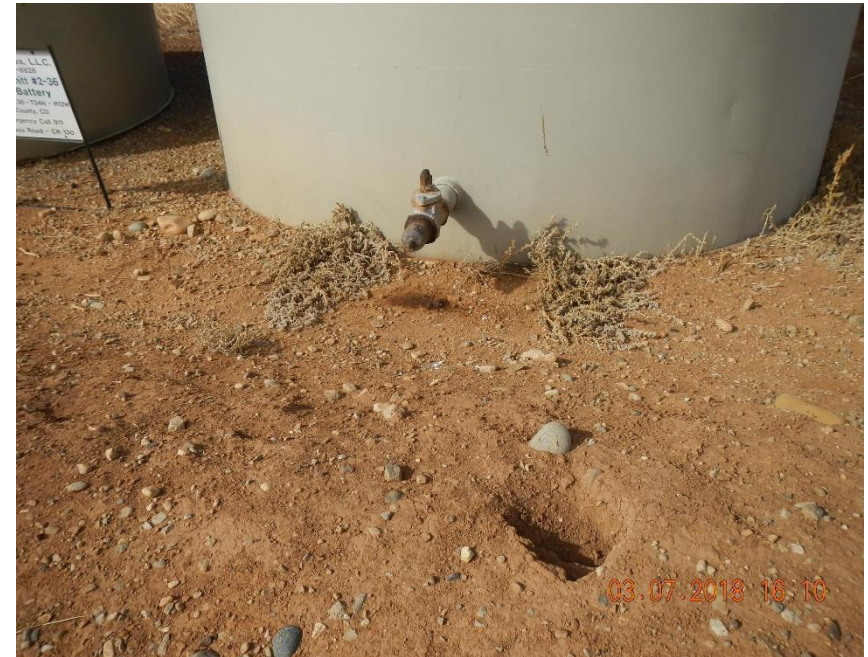
Stained soil below load out valve on eastern tank. Animal burrow in secondary containment berm.
