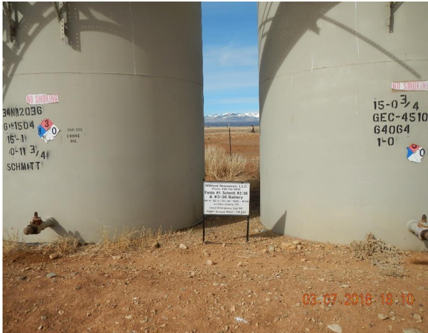
2 – 300 bbl. ASTs labeled crude oil at tank battery. Note stained soil below load out valves
