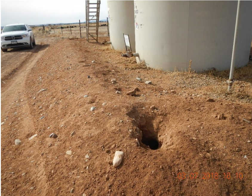
Animal burrow in secondary containment berm. Capacity of secondary containment does not appear to be adequate.
