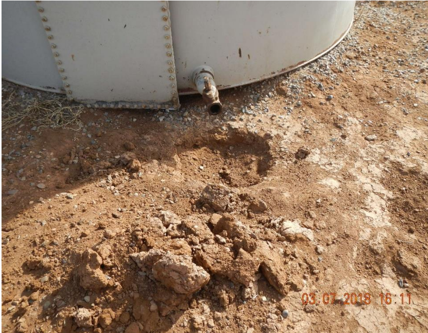
Soil below valve on western tank has been excavated.
