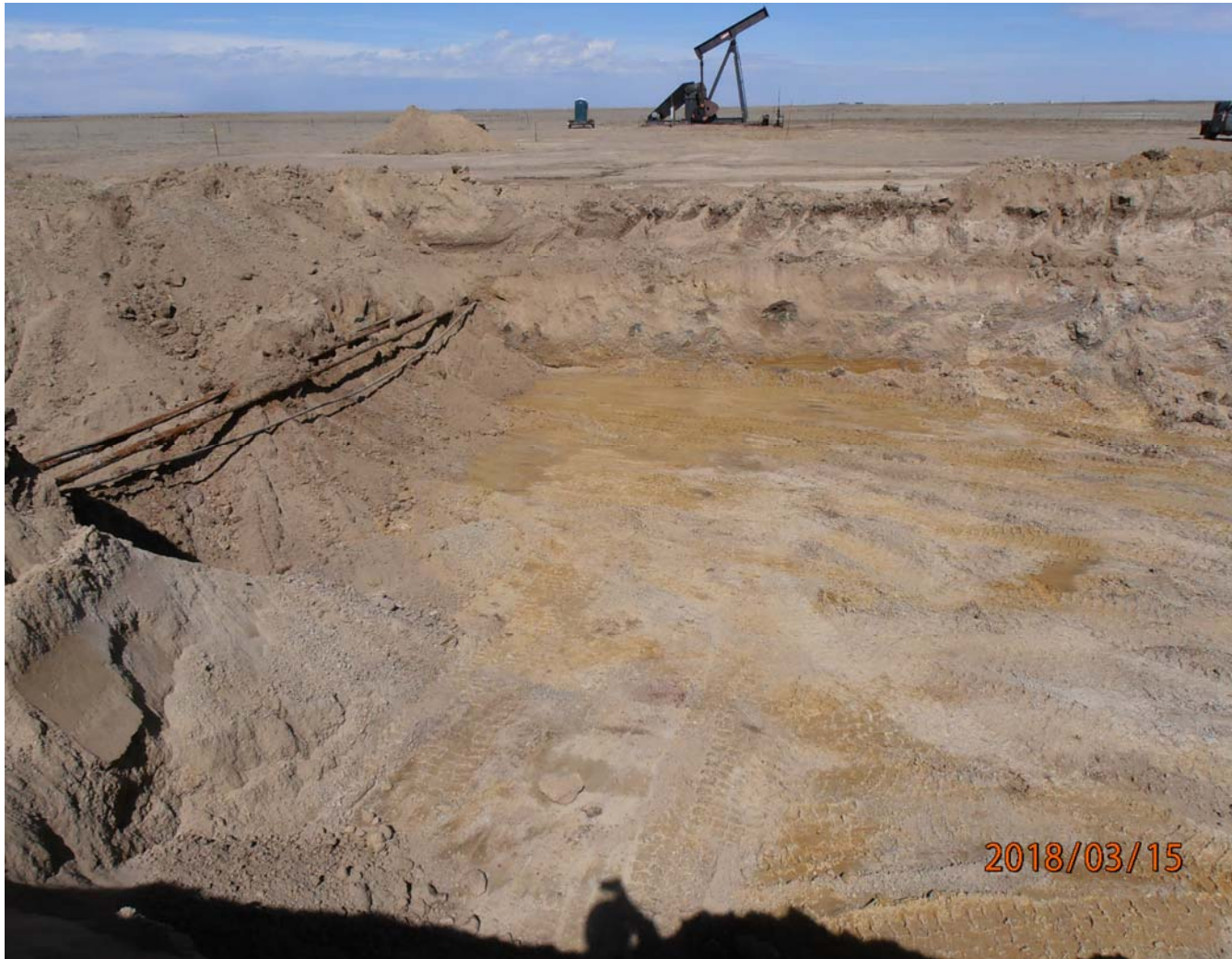
Photo 1 – Photo of excavation near source area viewing north. Croissant #4 in background. Flowlines on left of photo (west end of excavation). A removed injection line serving the Croissant #1 was present east of the flowlines.
