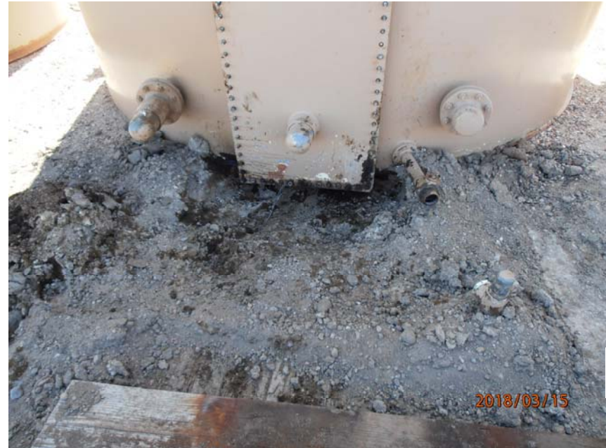
Photo 6 – North side of center crude oil AST. Oily material extends beneath tank.
