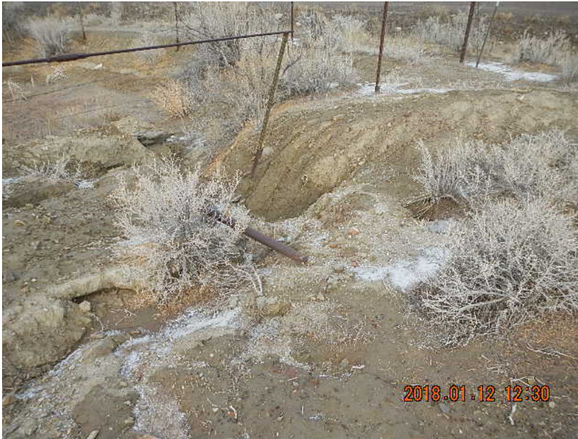
Erosion cuts into blow down pit
