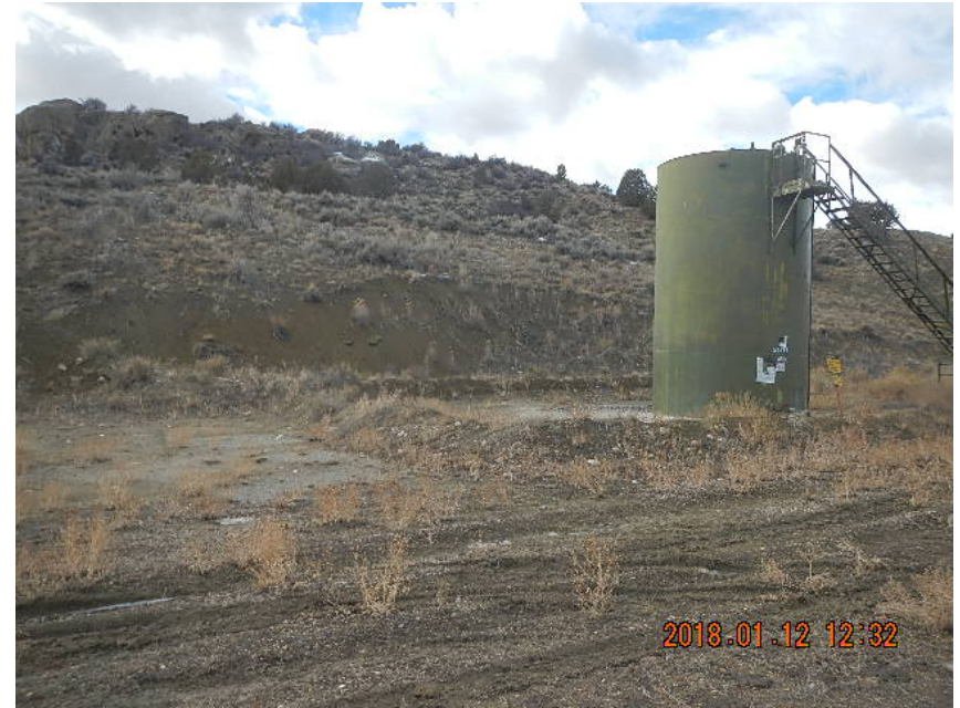
Slope not stable – erosion cuts
