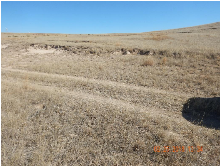
Photo 1: Photo taken from the south end of the location, facing northeast. Photo shows erosion and contouring concerns remain evident on the east and northeast ends of the location.
