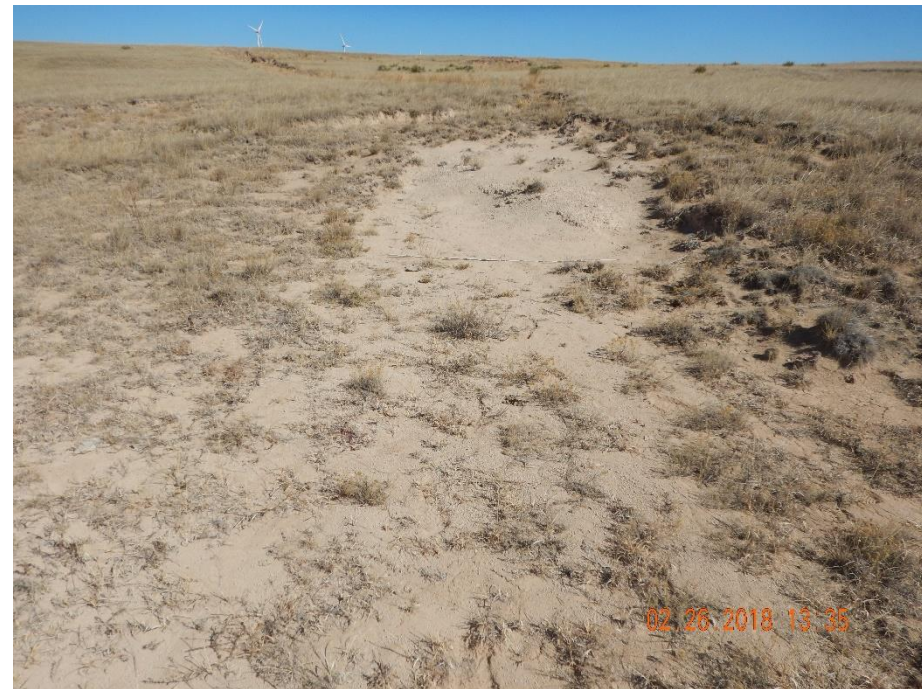
Photo 6: Photo taken from the east end of the location, facing northeast. Photo shows areas of the location where desirable perennial vegetation has failed to establish and stormwater erosion is causing degradation. These concerns appear to have been documented in previous inspections.
