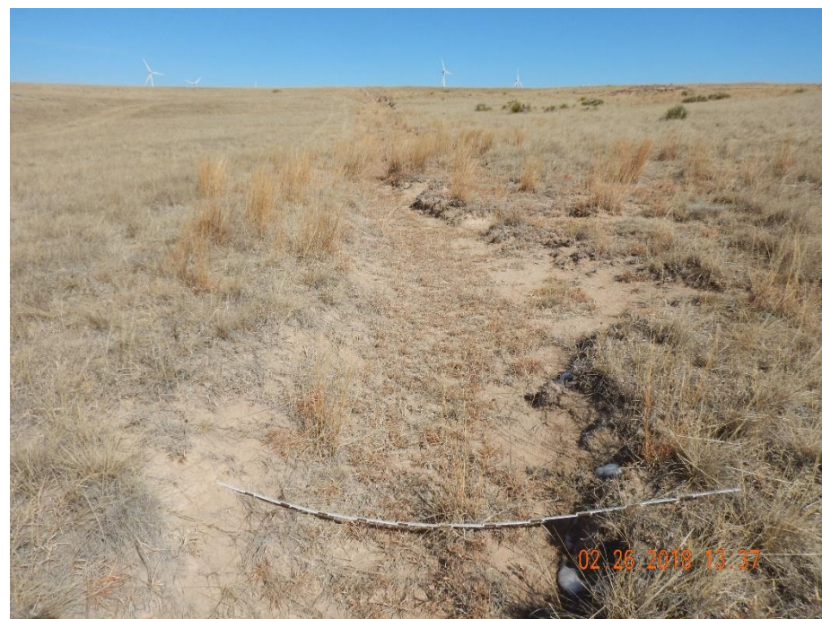
Photo 10: Photo taken from the access road on the northeast end of the location, facing north. Photo shows access road does not appear to have been adequately contoured and stabilized. Access road has acted as a channel for stormwater, allowing flows to concentrate and cause stormwater erosion degradation and incising to occur on both the access road and location. These concerns have been documented in previous inspections.
