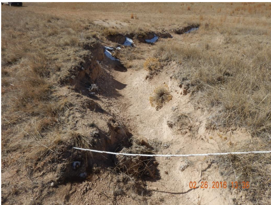
Photo 9: Photo taken from the northeast end of the location, facing west. Photo shows areas where stormwater runoff from the access road has eroded a large gully (see in photo 7) onto the location. 6 foot measuring stick for reference.
