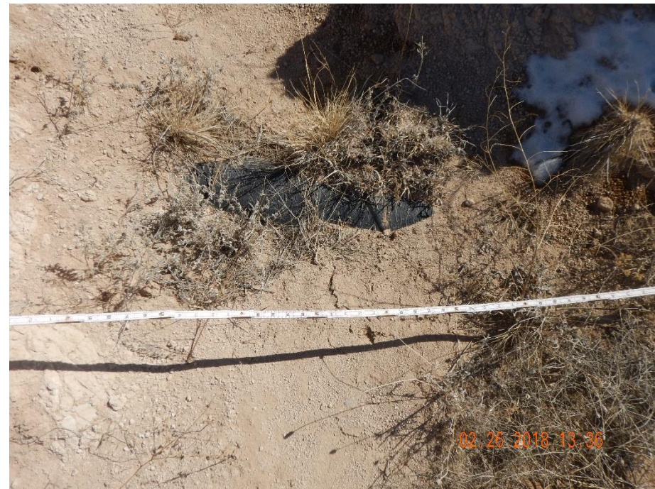
Photo 8: Photo taken from the erosion degradation observed on the northeast end of the location. Photo shows area of exposed pipeline likely revealed due to stormwater erosion
