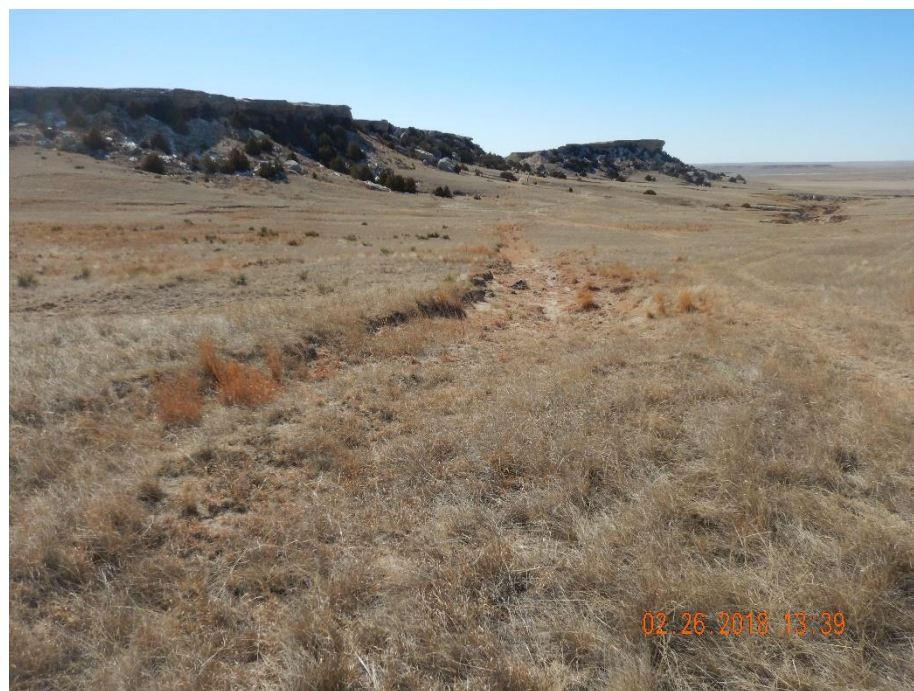
Photo 12: Photo taken from the access road, north of the location, facing south. Photo shows access road does not appear to have been adequately contoured and stabilized. Access road has acted as a channel for stormwater, allowing flows to concentrate and cause stormwater erosion degradation and incising to occur on both the access road and location.
