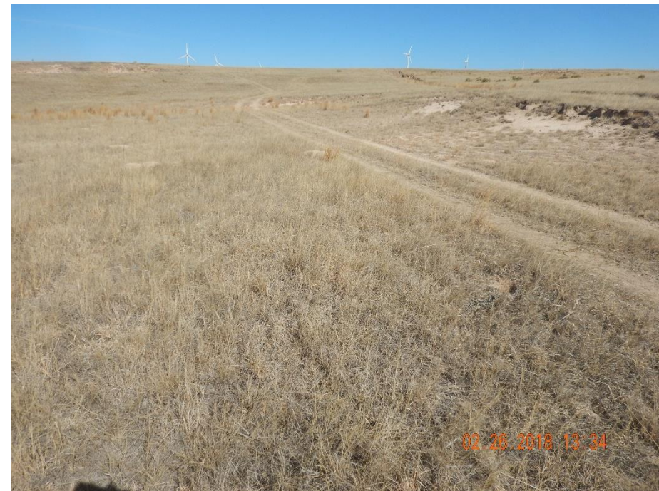
Photo 2: Photo taken from the south end of the location, facing northeast. Photo shows erosion and contouring concerns remain evident on the east and northeast ends of the location. Two-track road seen in photo is not the historic access road and appears to have been created relatively recently based on historic imagery.
