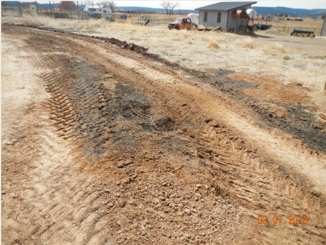
Photo 5. View of unknown black material within the western portion of the project area, covers an area that is approximately 50 feet long and 15 feet wide, and seeping westward off of the project area.
