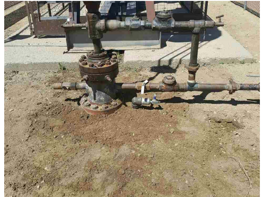
Photo from operator showing bradenhead plumbed to surface.
