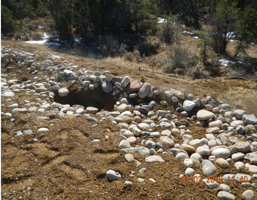
Storm water BMP in disrepair.
