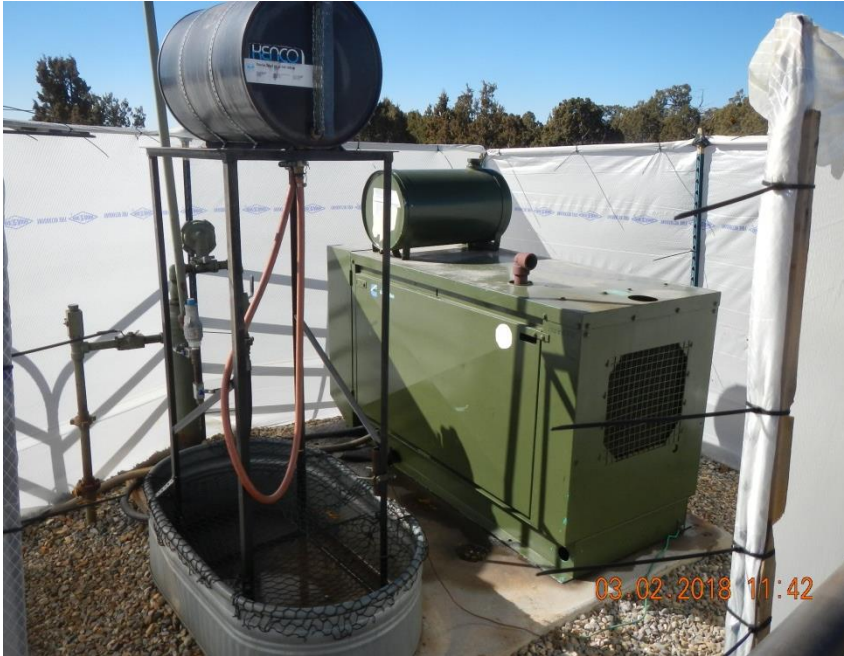
Lube oil container with secondary containment and leaking generator.
