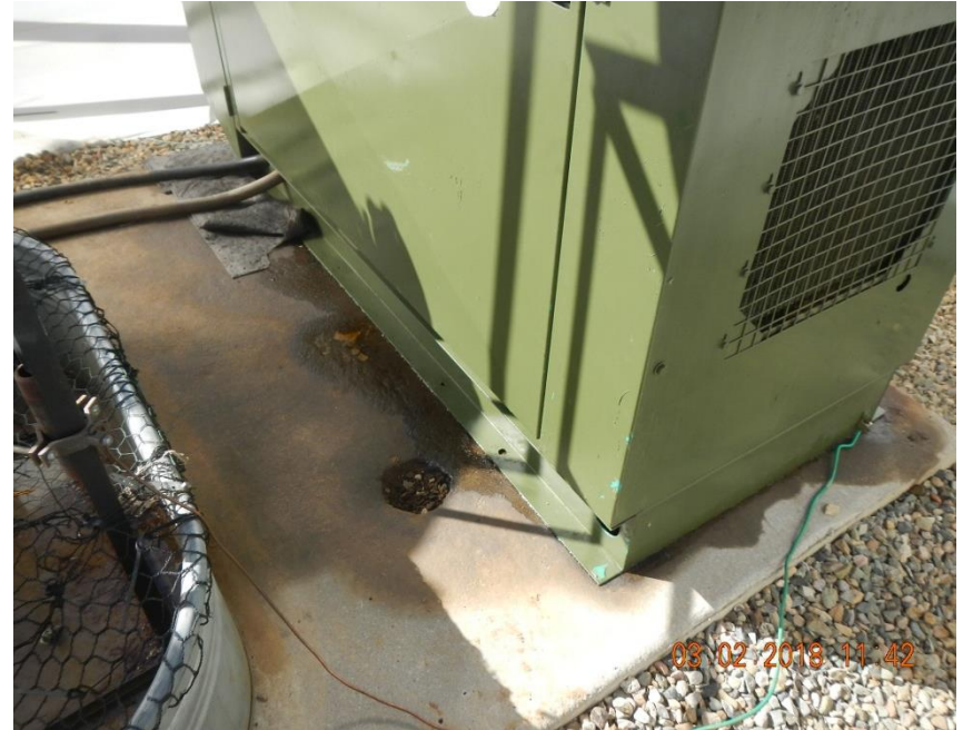
Lube oil leaking from equipment.
