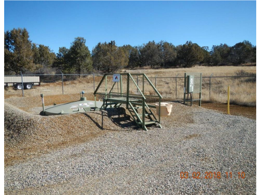
PBV with drip pot on load out line.
