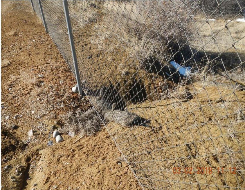
Wattles in erosion channel on western edge of location.
