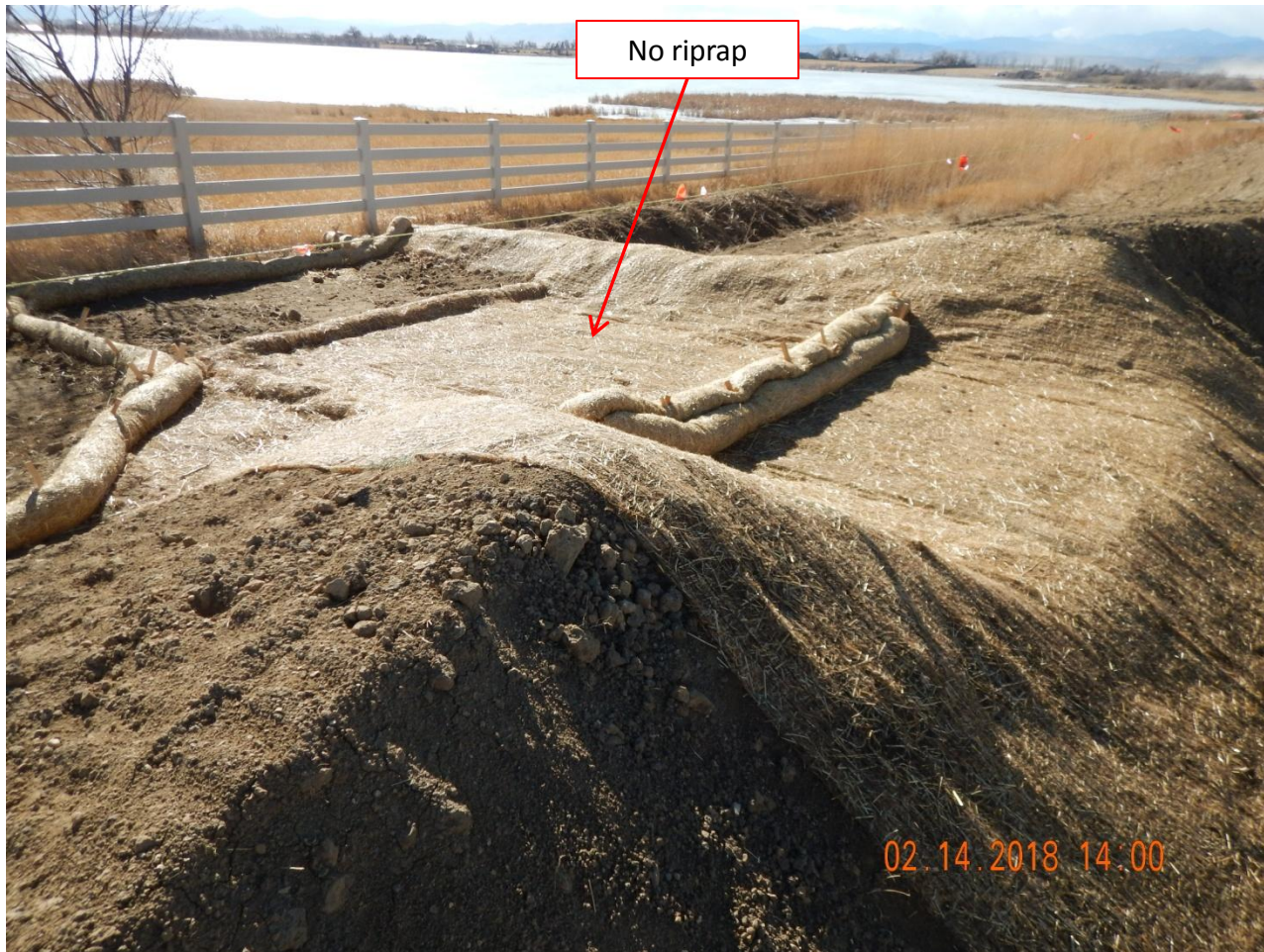
Photo 4. Photo taken from the southeast sediment basin spillway, facing Southwest. See comments under Photo 2.
