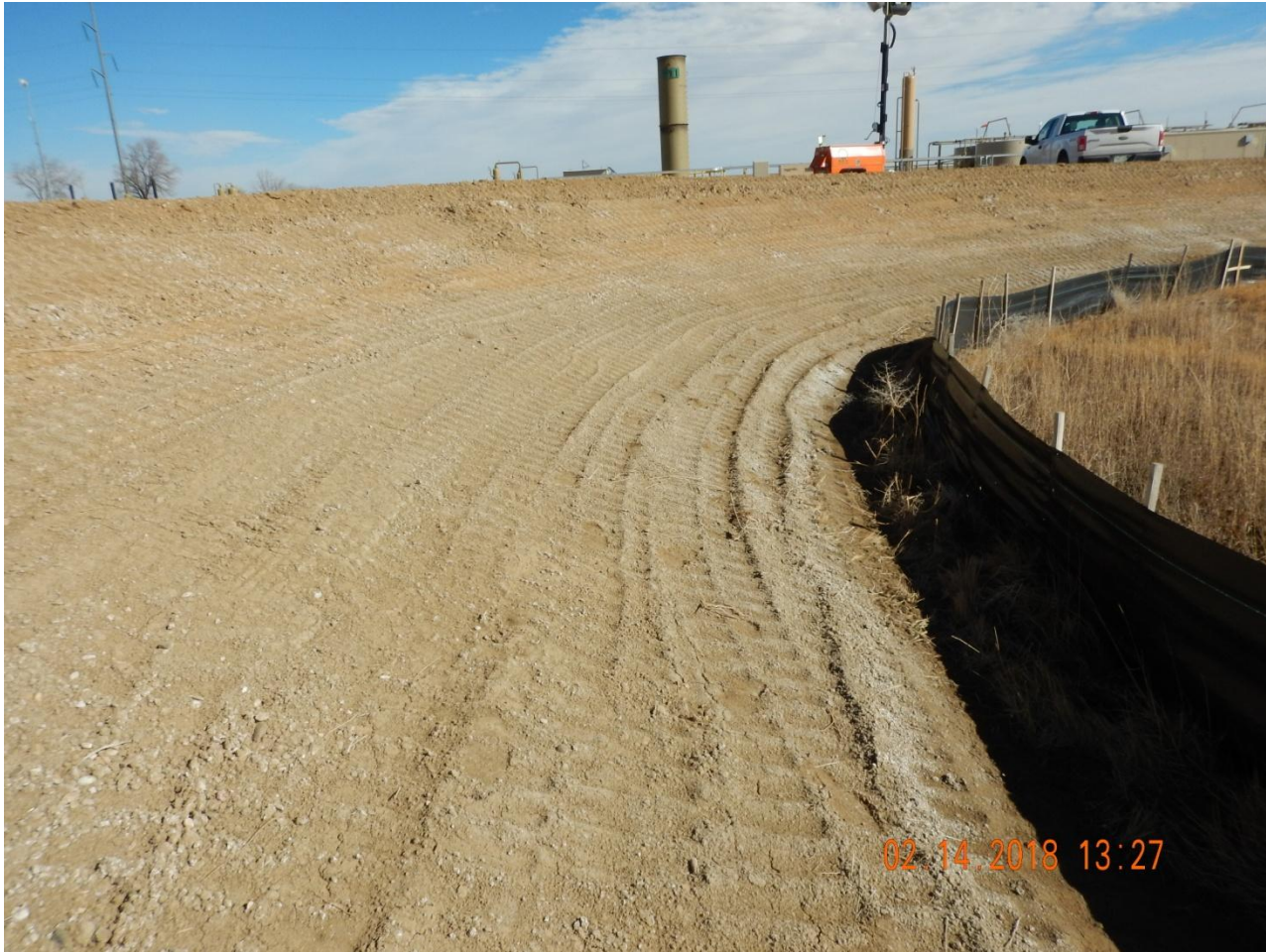
Photo 10. Photo taken from the western location, facing East. Operator has improperly tracked the western side slopes. Equipment tracking should be tracked perpendicular to the slope.
