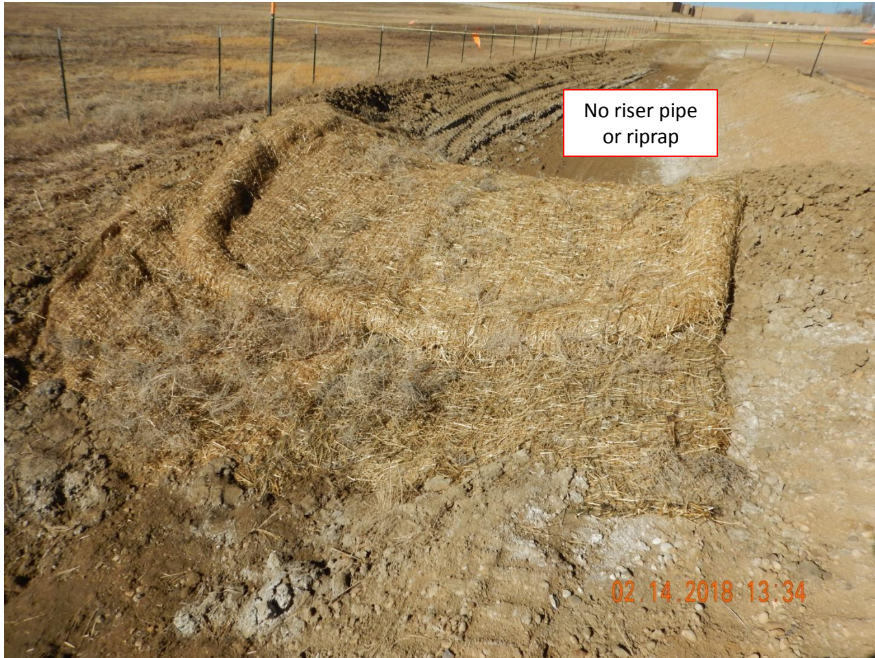
Photo 2. Photo taken from the western sediment basin spillway, facing North. See comments under Photo 1. Operator has not installed a riser pipe and the spillway has not been constructed with riprap.
