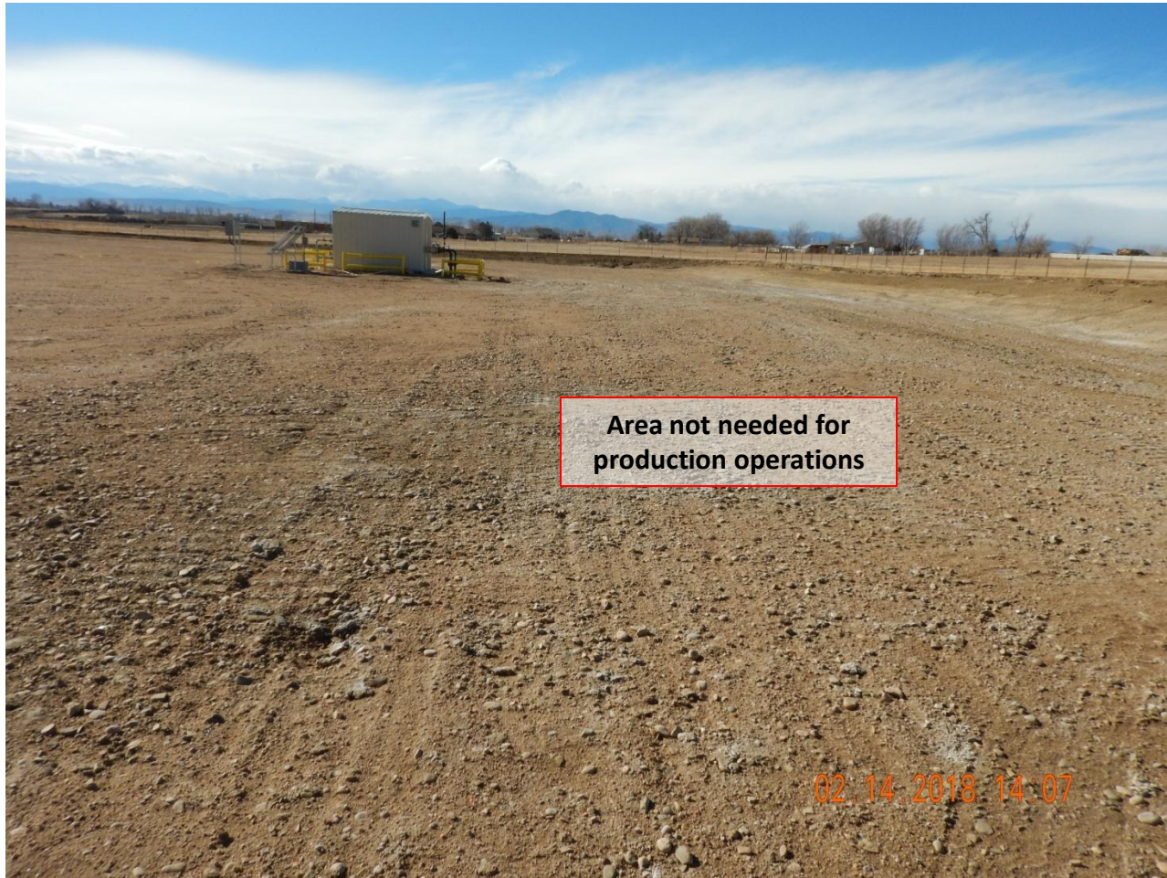
Photo 7. Photo taken from the northeastern location, facing West. Operator has failed to perform interim reclamation per Rule 1003.
