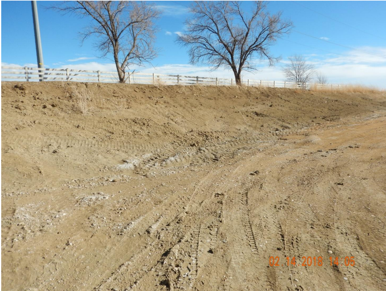
Photo 6. Photo taken from the northeastern location, facing East. Operator has not properly stabilized the cut slope which is susceptible to erosion.
