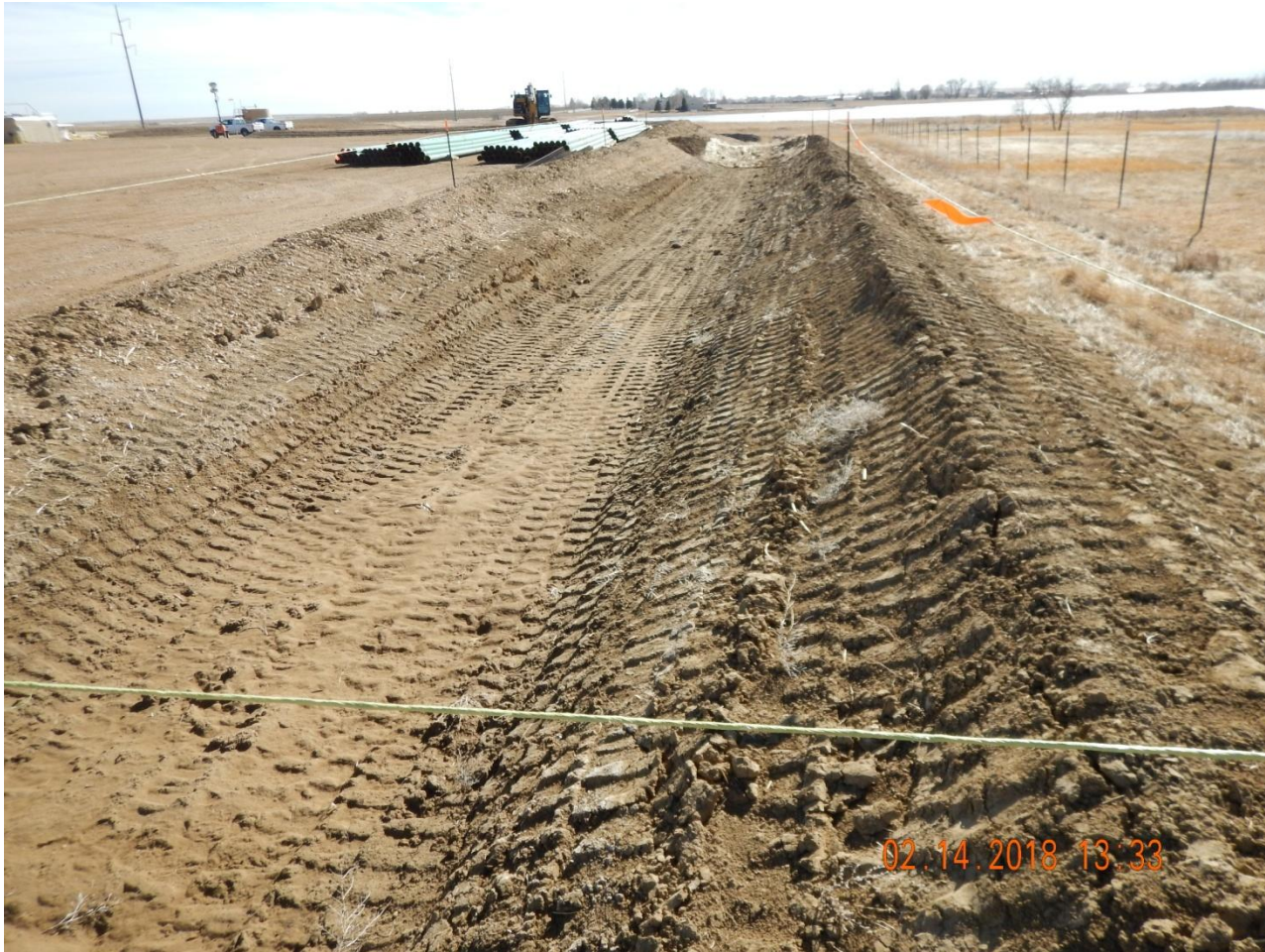
Photo 1. Photo taken from the western sediment basin, facing South. Operator has installed a sediment basin increasing the sediment storage area. However, Operator has not constructed to the sediment basin per the Stormwater Technical Drainage Analysis Memo.
