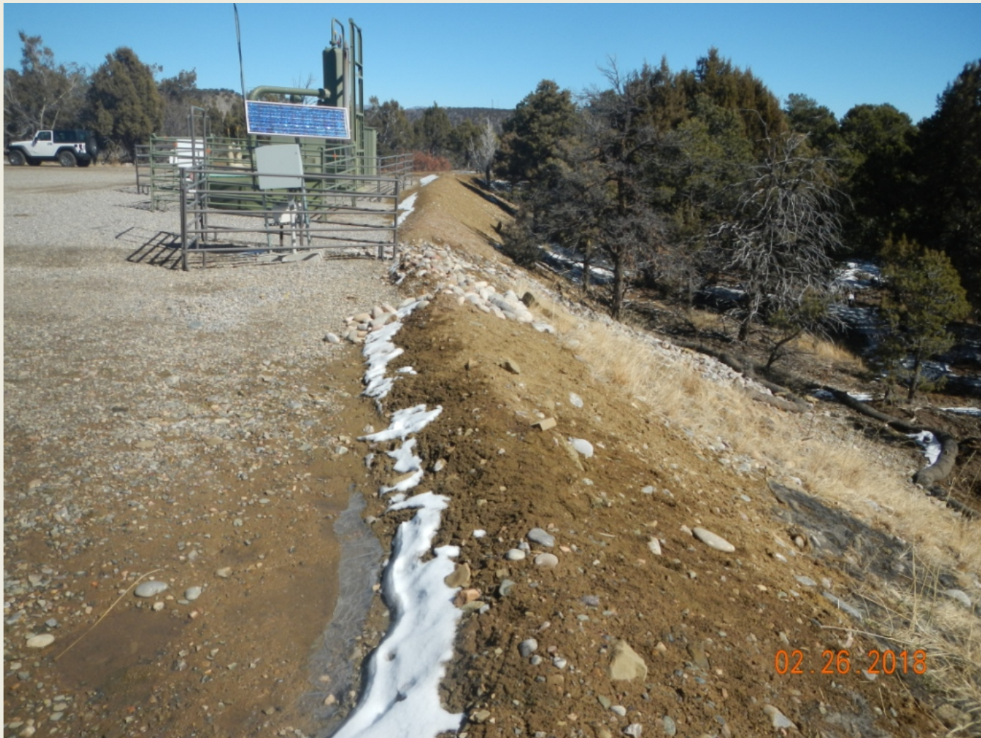
Photo 3. View of the southern portion of the project area from the southwestern corner facing eastward. Poor revegetation on berms and fill slopes. These should be seeded in spring 2018.
