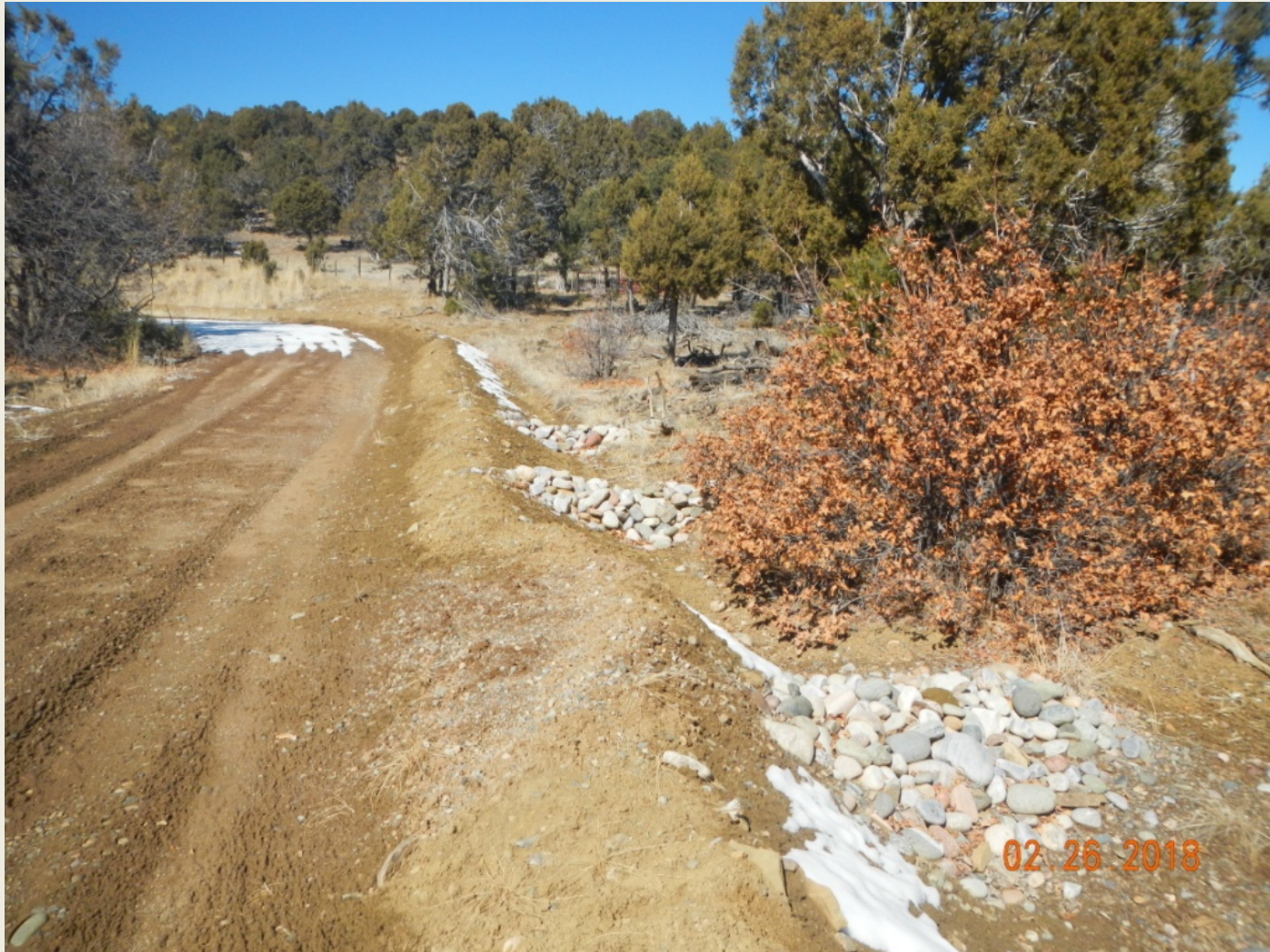
Photo 4. View of stormwater controls in the eastern portion of the project area facing northward. Appear to be functioning at this time .
