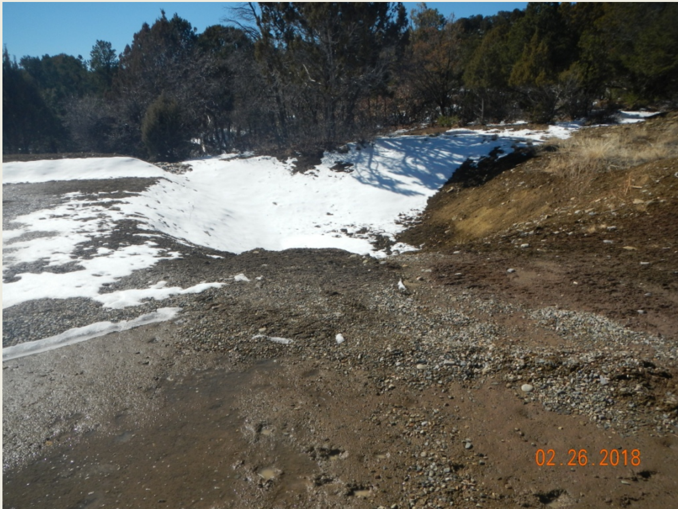
Photo 5. View of silt trap in the northwestern portion of the project area, appears to functioning at this time.
