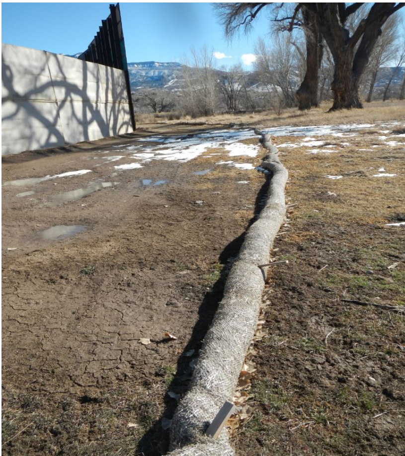
Photo#5: Wattles installed along West Track.
