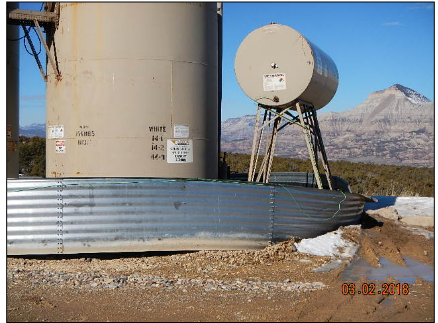
Photo 4. Damaged tank containment.
