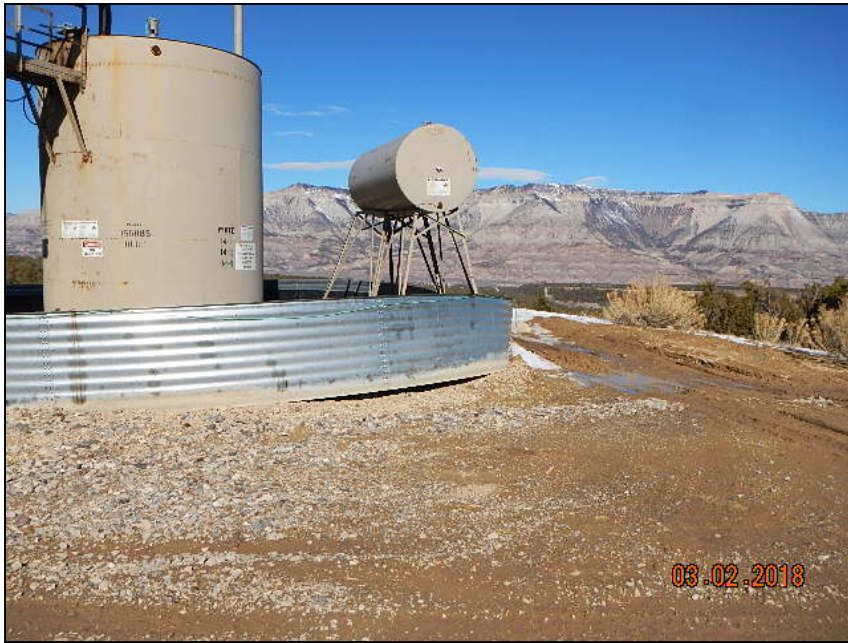
Photo 3. Damaged tank containment.
