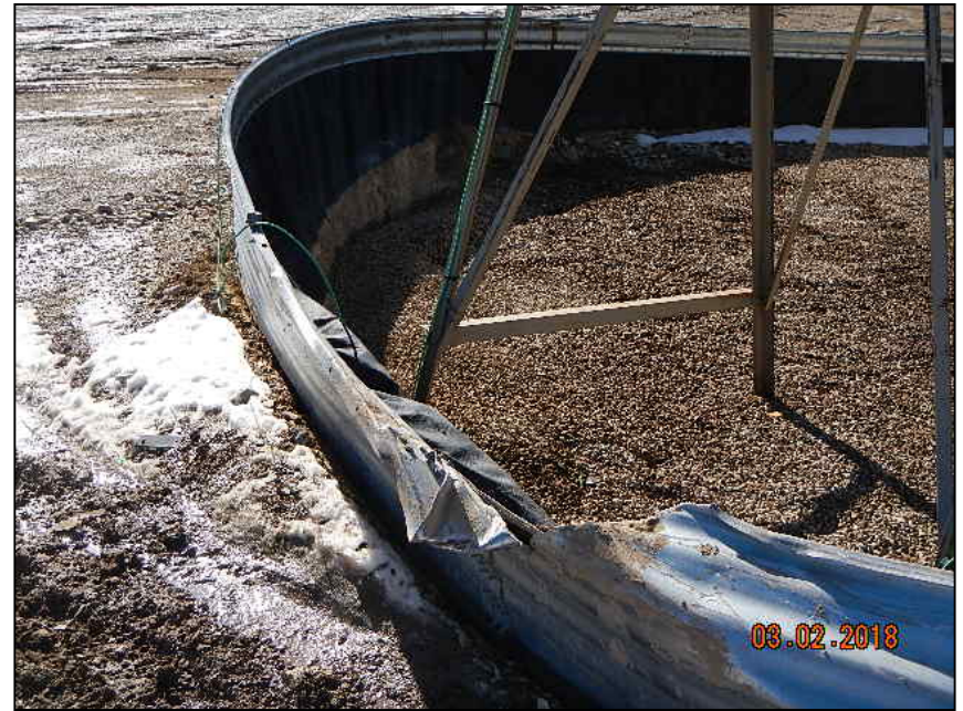
Photo 2. Damaged tank containment.
