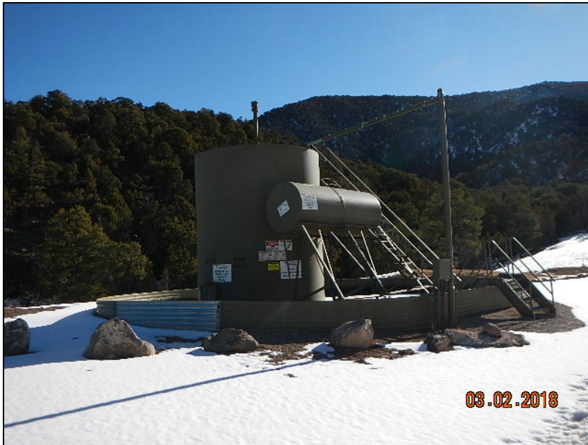
Photo 1. Methanol tank is tipped over against 300bbl tank.
