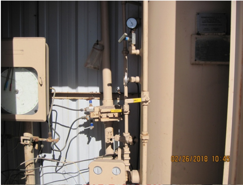
3. Meter run and vertical gas separator
