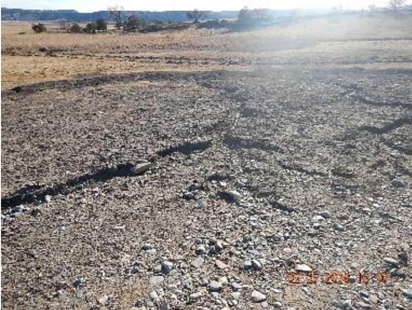
Photo 5: Erosion channels on SW fill slope.
