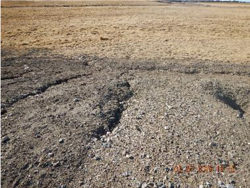
Photo 7: Erosion channel on W and NW fill slope.
