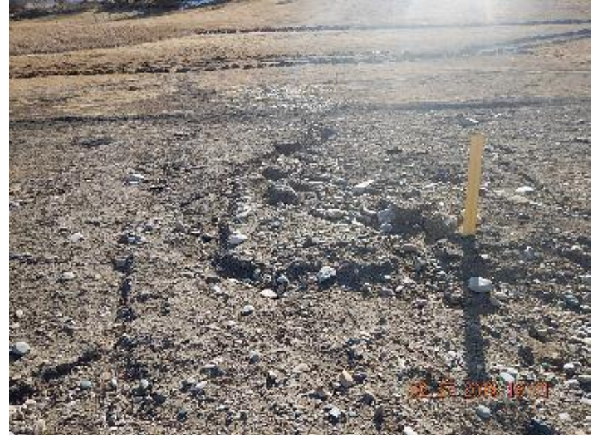
Photo 6: Erosion channel on W fill slope.
