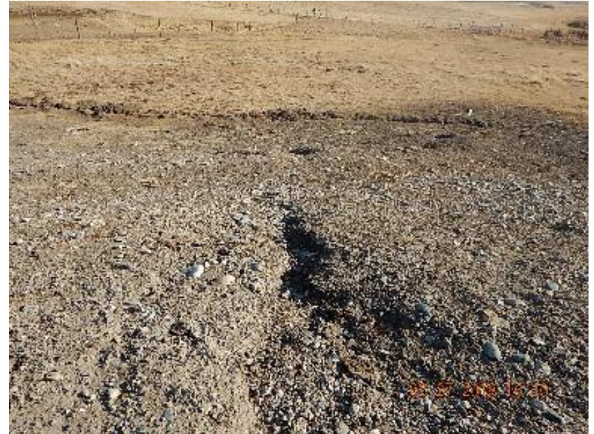
Photo 4: Erosion channel on SW fill slope.
