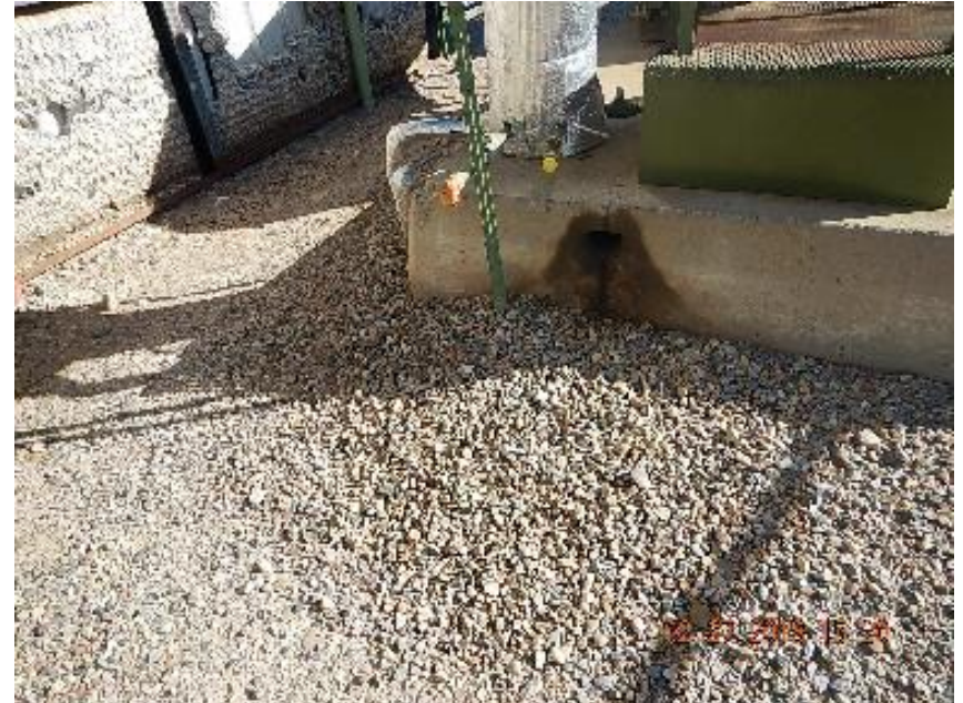
Photo 8: Cleaned up impacted soil and gravel.
