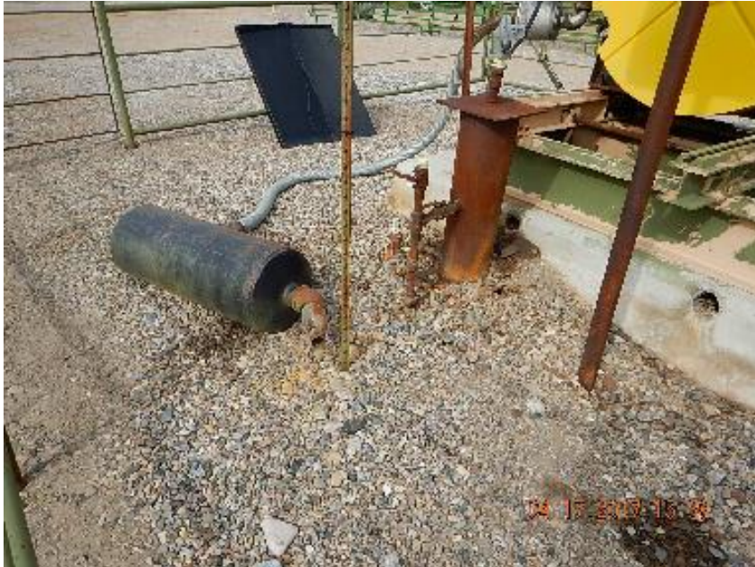
Photo 5: Stained soil at the muffler, ground behind lube oil tank, and supply gas knock out for the Squires 3 previous inspection
