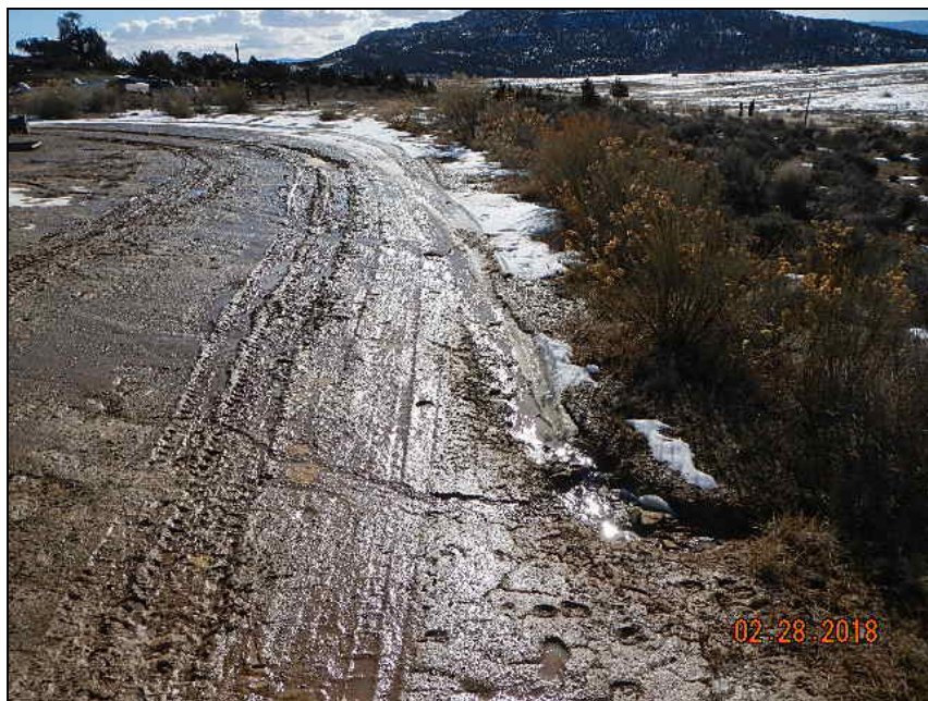
Photo 3. Erosion on access road.
