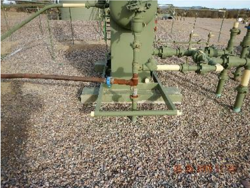
Photo 5: Unused riser at #1A separator.
