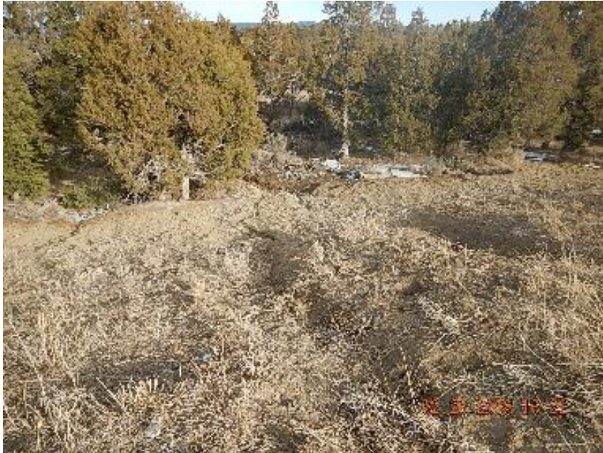
Photo 9: Erosion channels and damaged waddles on E fill slope.
