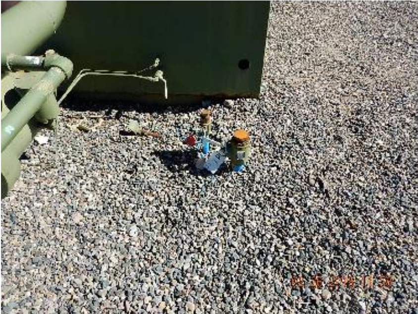
Photo 7: Unused risers at 15-4 separator.
