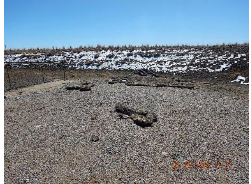
Photo 8: Damaged waddles.
