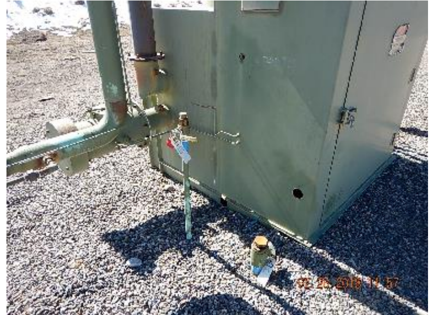
Photo 6: Unused 1" riser at 15-2 separator.
