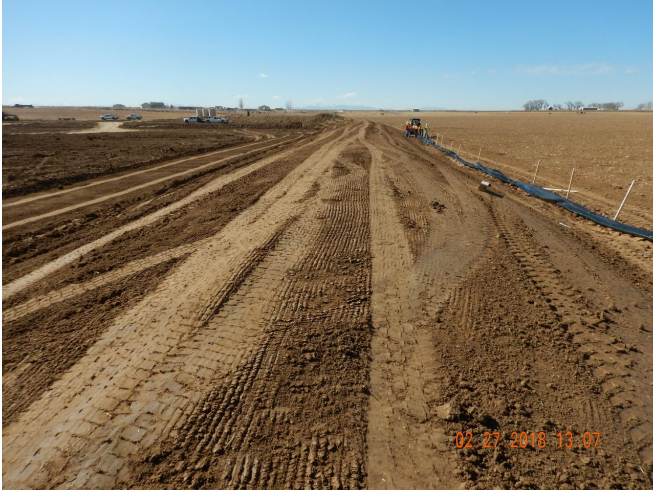
Photo 7. Photo taken from the northeastern location, facing West. Photo illustrates the topsoil stockpile that has been salvaged and stored along the northern and a portion of the western location.
