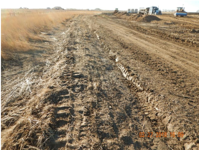
Photo 3. Photo taken from the southern location, facing West. Appears the Operator has further stabilized the berm BMP with equipment tracking. Operator was in-process of installing a silt fence BMP around the entire location during this inspection.
