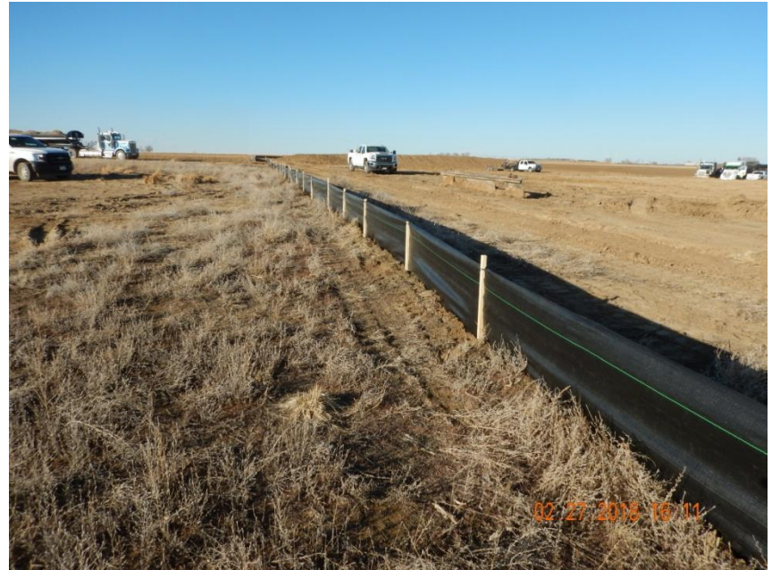
Photo 4. Photo taken from the southwestern location, facing North. Photo illustrates the Operator has installed a silt fence BMP around the western location.
