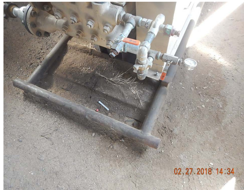
Photo 4: Stained soil at injection pump
