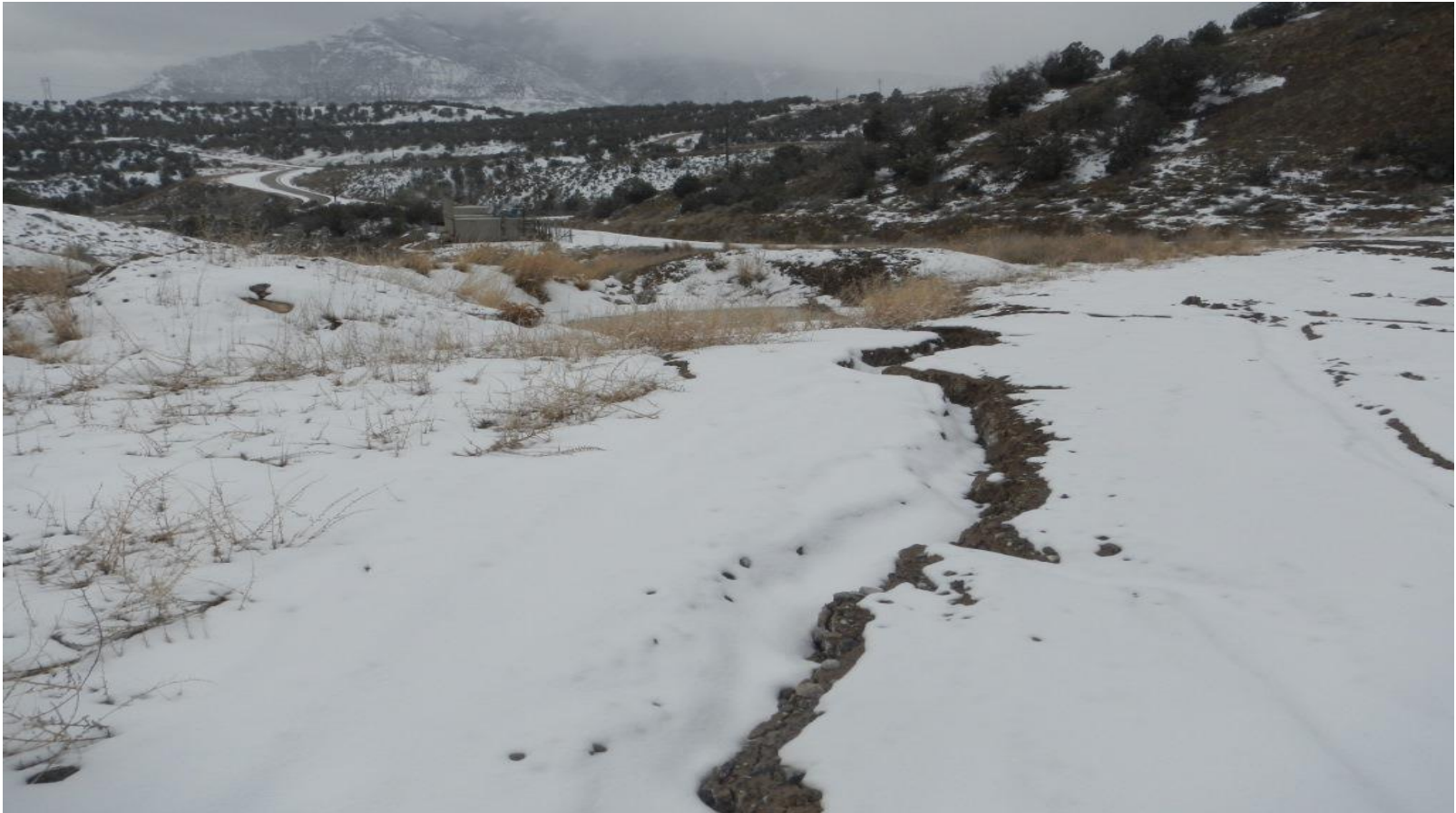
Photo#2: Erosion of Pad Surface is occurring on Southeast side of Location.
