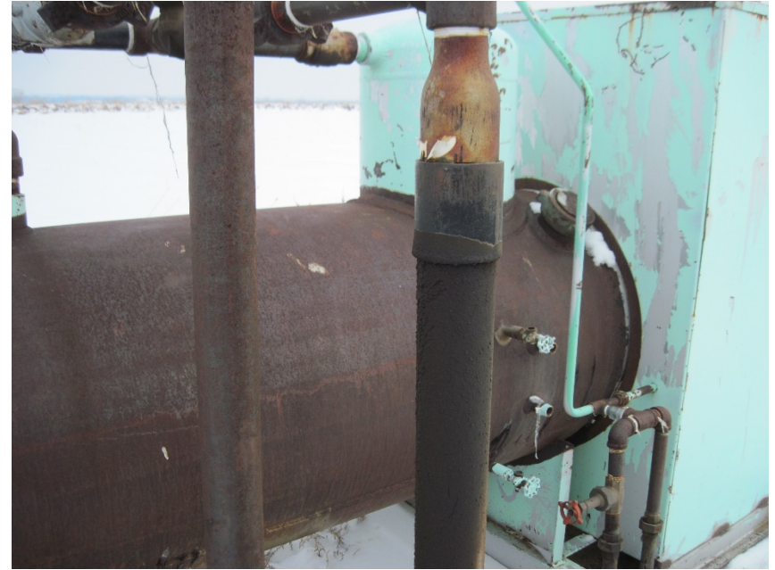
3" PIPE LEAKING AT SWEDGE
