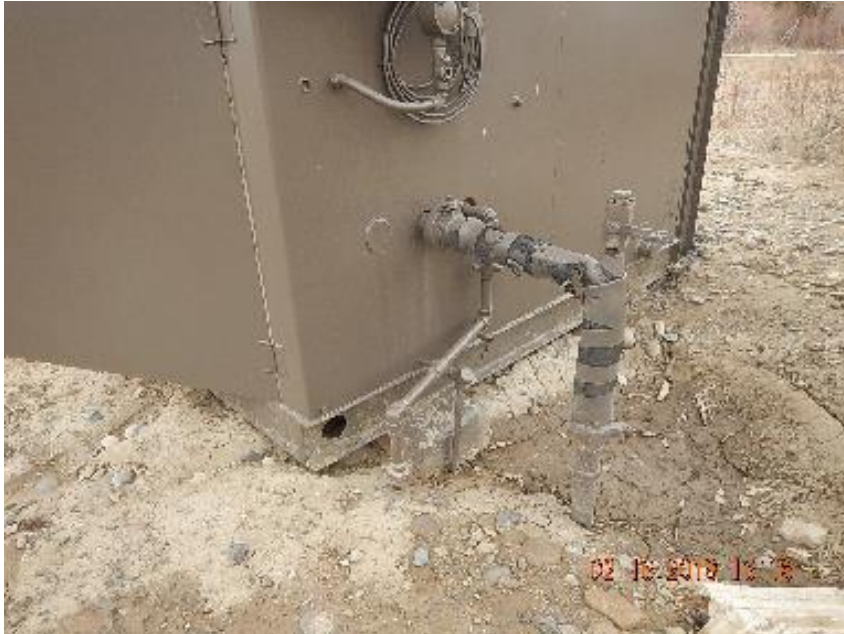
Photo 3: Connected steel 1" supply gas line at separator.
