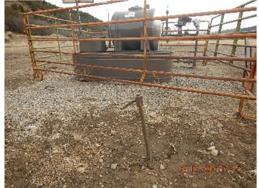
Photo 2: Steel 1" riser outside wellhead fencing.
