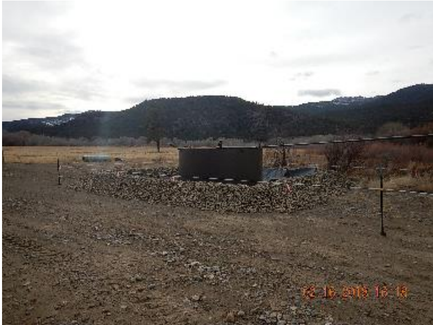
Photo 5: Produced water open top with no labels/sign.
