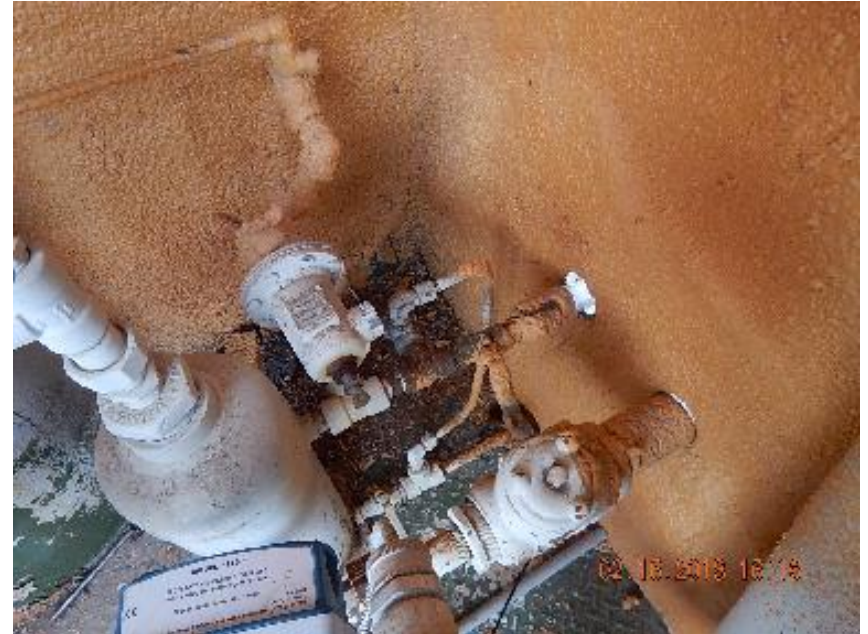
Photo 4: Connected 1" steel supply gas line inside separator.
