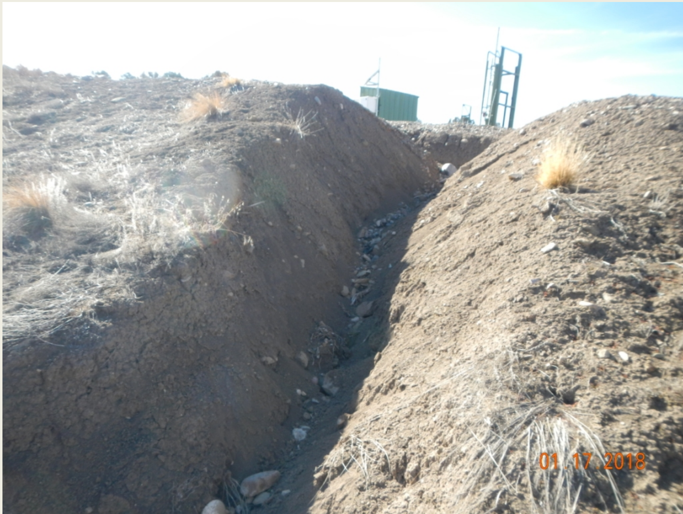
Photo 5. View of another erosional channel approximately 5 feet wide and deep in the eastern portion of the project area. Stabilization measures are needed here.
