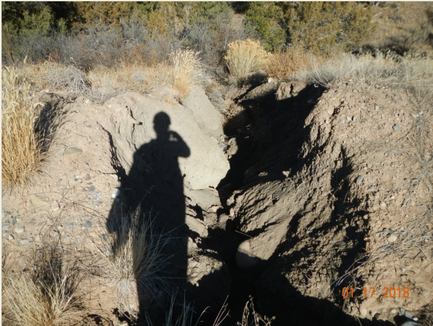
Photo 4. View of an erosional channel approximately 5.5 feet wide and deep in the northern portion of the project area. Stabilization measures are needed here.
