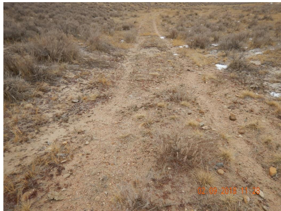
Photo 10: Photos 10-15 taken from the access road. Photos shows access road does not meet reclamation standards. Gravel/ruts evident. Road has not achieved a uniform desirable perennial vegetative cover.
