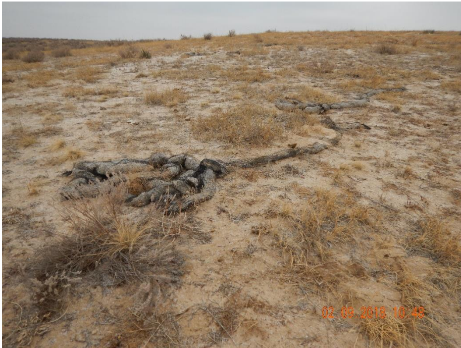
Photo 1: Photo taken from the west end of the location, facing north. Photo shows stormwater and sediment control BMPs (wattles) that have not been maintained, are no longer in proper functioning condition, and is considered debris. Wattle debris was observed on the northern, northwestern and southern ends of the location.
