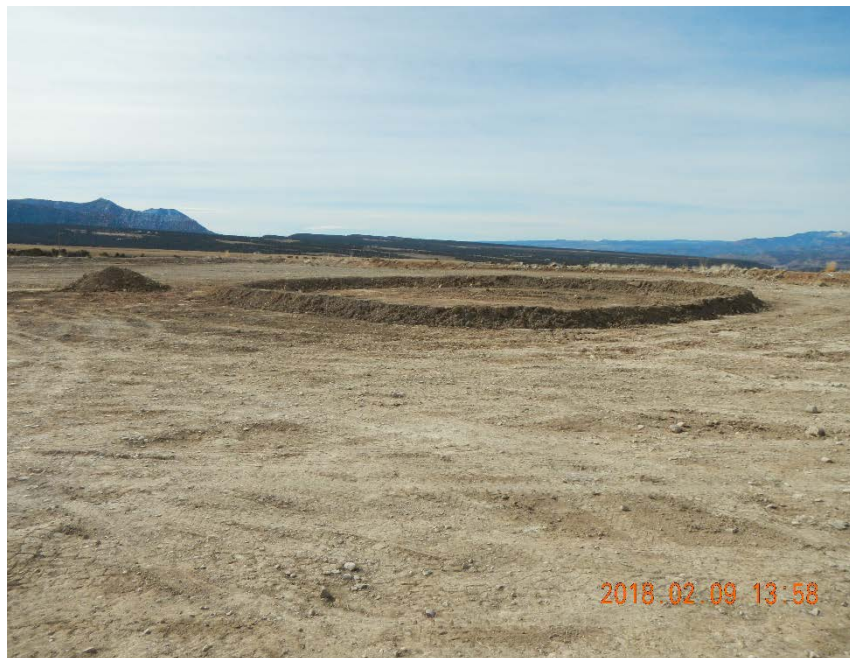
Location where the tank was being torn down. Circular berm contained spilled sludge. There is a small stock pile on the left side of the berm.
