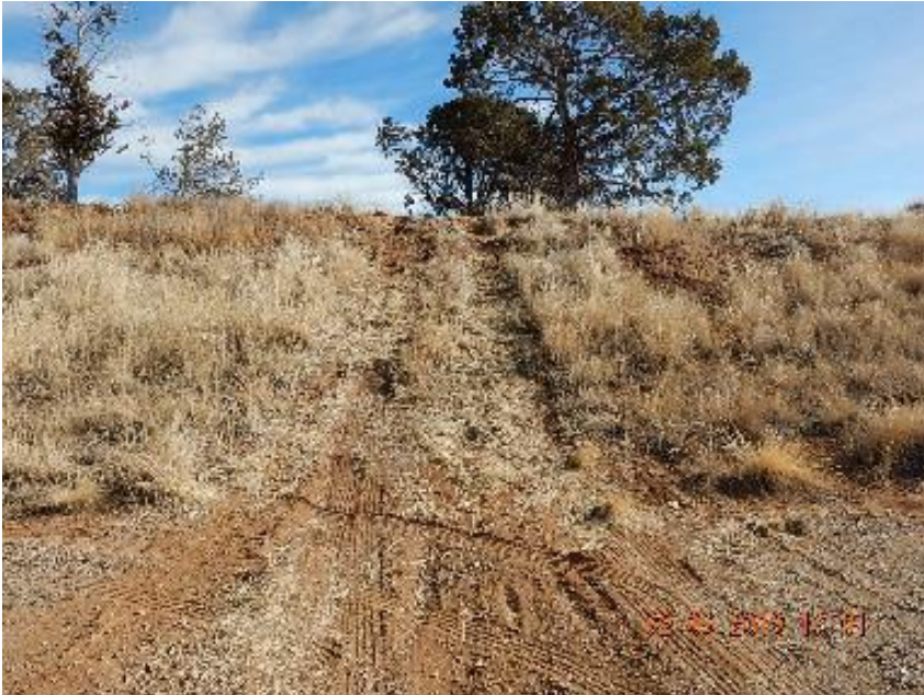
Photo 5: Vehicle tracking on cut slope.
