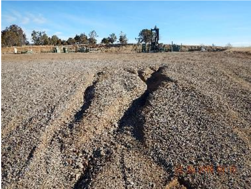
Photo 3: Erosion channel at entrance.
