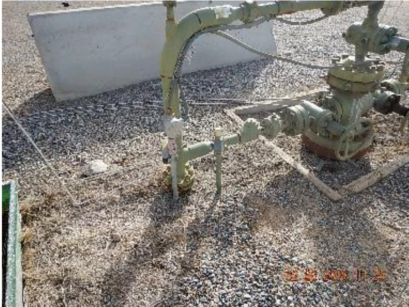
Photo 7: Unused 1" supply gas line at the #1 – A wellhead.
