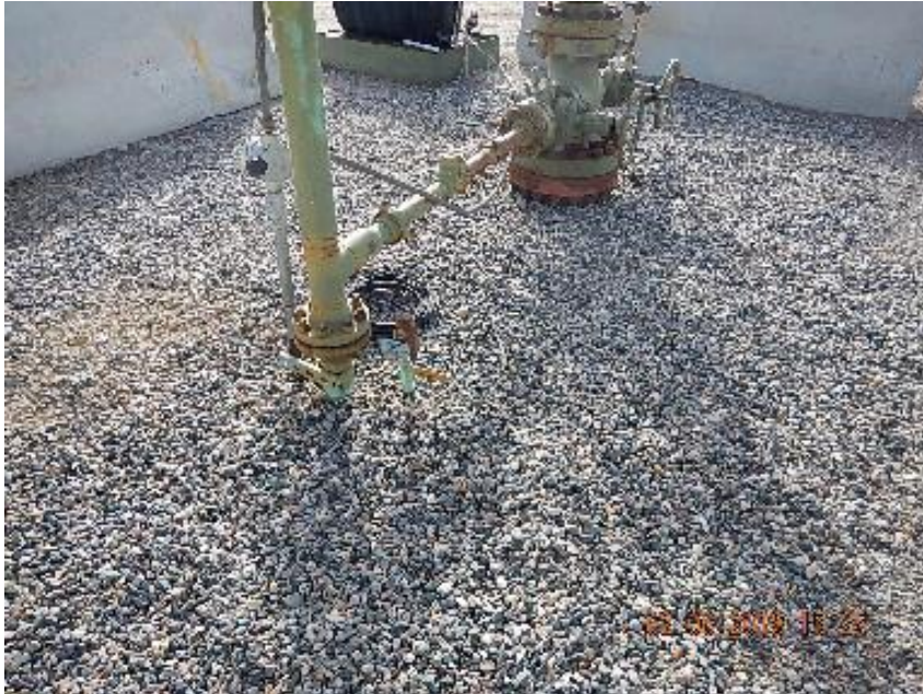
Photo 3: Unused 1" supply gas line at the #2 – A wellhead.
