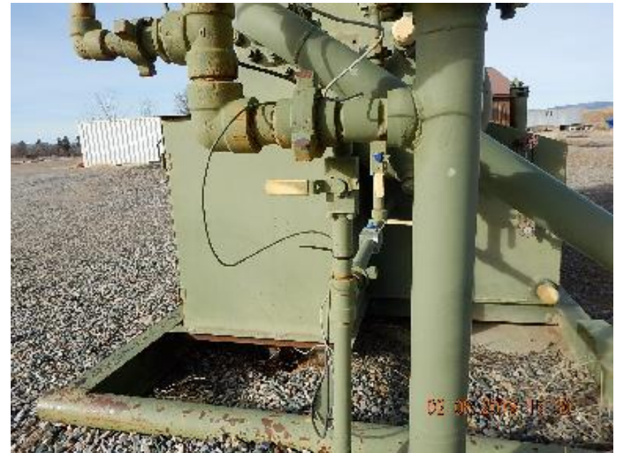
Photo 6: Unused 1" supply gas line at the #1 – A separator.
