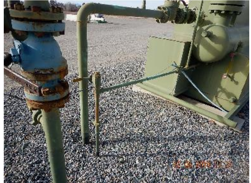
Photo 2: Unused 1" supply gas line at the #2 – A separator.
