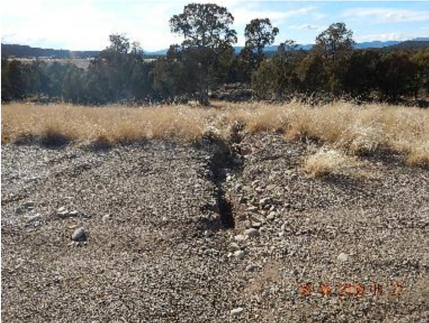
Photo 7: Stormwater erosion channel off W edge of location.
