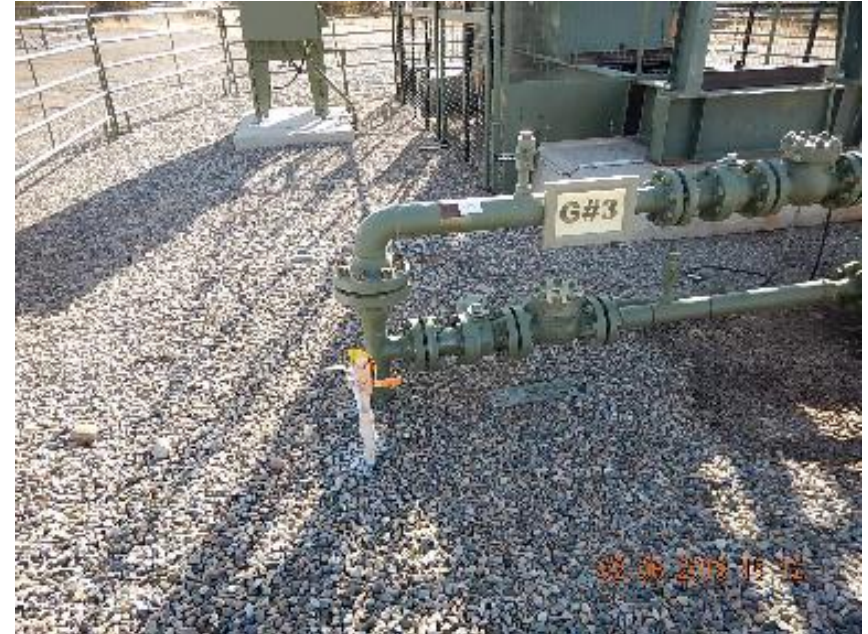
Photo 4: Unused supply gas riser at G#3 wellhead.
