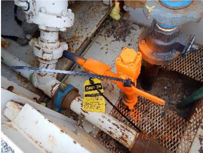
Photo 5: Unused supply gas riser inside G#3 separator cabinet.
