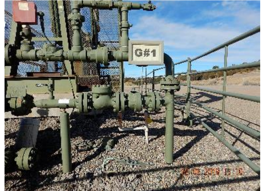
Photo 2: Unused supply gas riser at G#1 wellhead.
