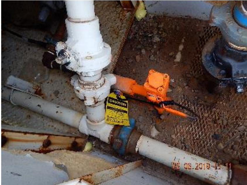
Photo 3: G#1 supply gas riser inside separator cabinet.
