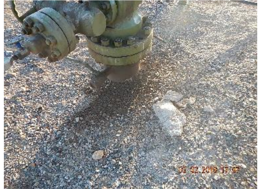
Photo 2: Impacted soil and gravel around base of wellhead.
