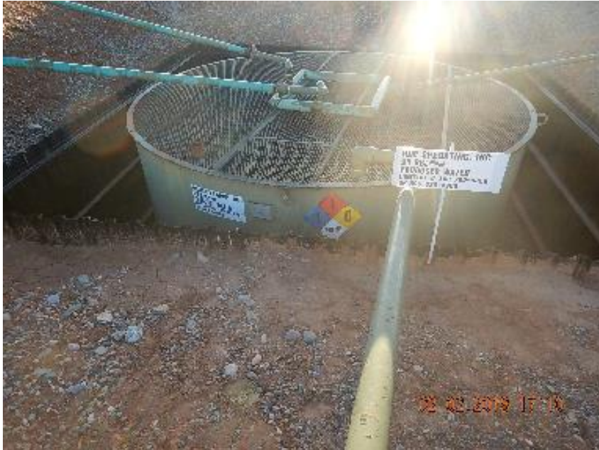
Photo 5: Open top tank with below and above grade labeling.
