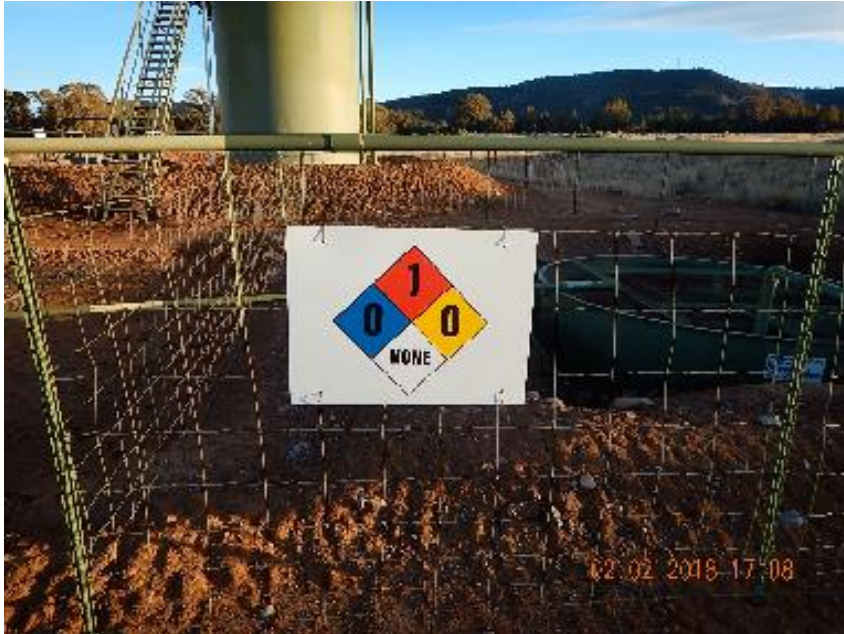
Photo 3: NFPA sign does not match NFPA labels on tanks.
