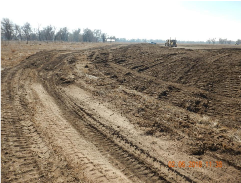
Photo 7. Photo taken from the northeastern location, facing South. Appears the Operator has salvaged and stored topsoil along portions of the northern and eastern location perimeter.
