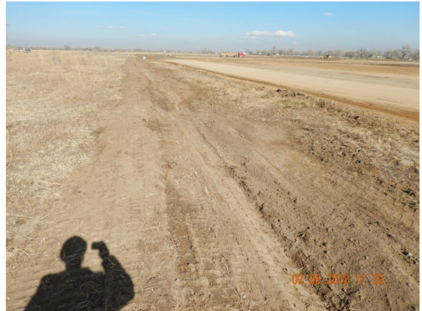
Photo 2. Photo taken from the western location, facing North. Ditch and berm BMP installed.
