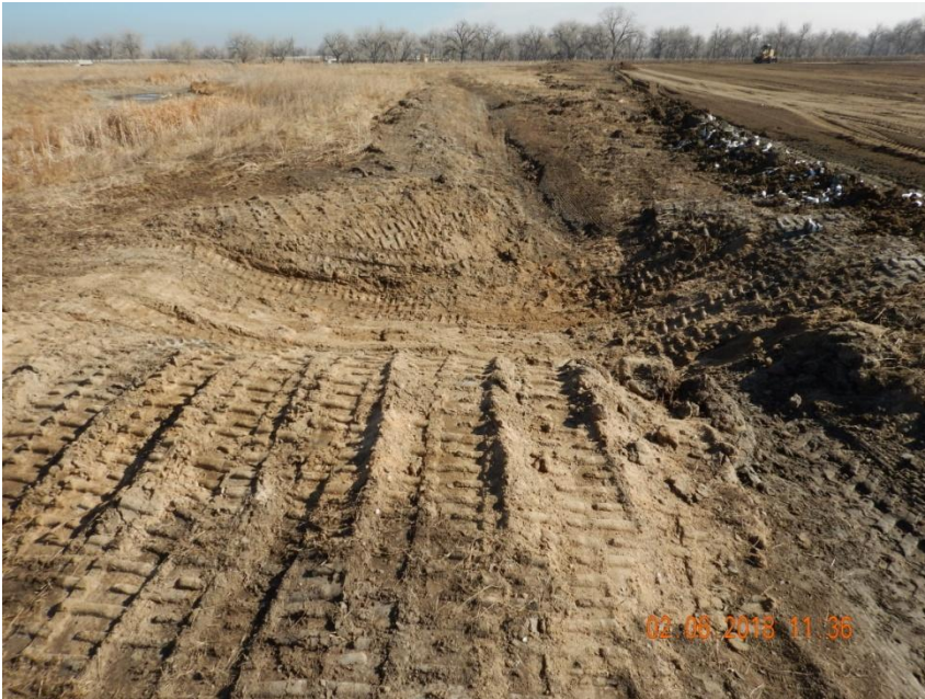
Photo 5. Photo taken from the northwestern location, facing East. Operator IN-PROCESS of constructing what appears to be a sediment trap.
