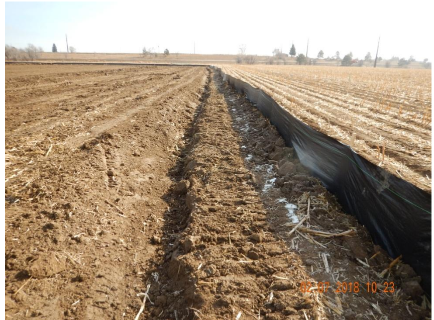
Photo 2. Photo taken from the southern location perimeter, facing South. Operator has installed a silt fence BMP around the entire perimeter of the location but the silt fence BMP has not been properly installed. A ditch BMP has been installed around the entire perimeter, inside of the silt fence BMP, but has not been installed in accordance with good engineering practices. Appears frozen soil conditions may have resulted in poor installation for both BMPs.
