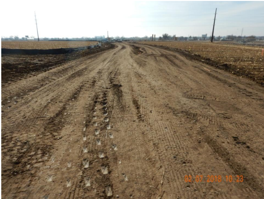
Photo 1. Photo taken from the southern location of the main access road, facing South. Operator has installed a silt fence BMP around the eastern portion of the access road.
