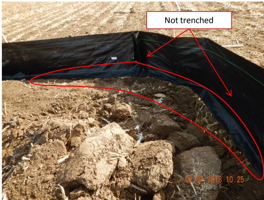
Photo 3. Photo taken from the southeast location perimeter on February 7, 2018, facing East. Operator has not properly trenched the silt fence BMP.
