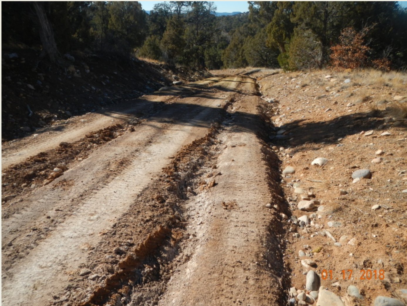
Photo 5. View of erosion occurring where concentrated stormwater flows down the access road creating erosional channels. Stormwater controls are needed.
