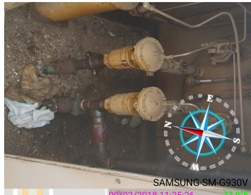
Stained soil and leaks in Dog House and trash in Dog House
